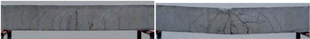
(a) Crack pattern for Beam Case I with at a drop-height of 0.3 m. (b) Crack pattern for Beam Case I with at a drop-height of 1.2 m.
