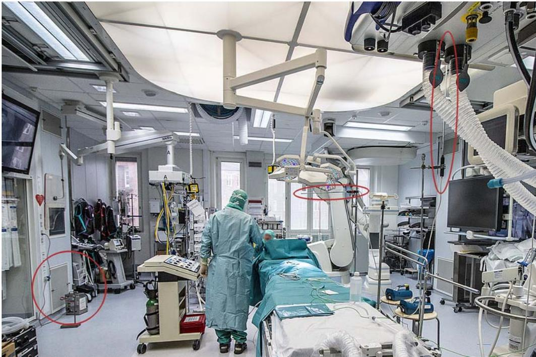
*Figure 26 Placing of particle counters in operating theatre. Red circle marks the counter at the exhaust ventilation, red horizontal oval marks the counter above operating bed and red vertical oval marks the counter measuring at the supply air.*
