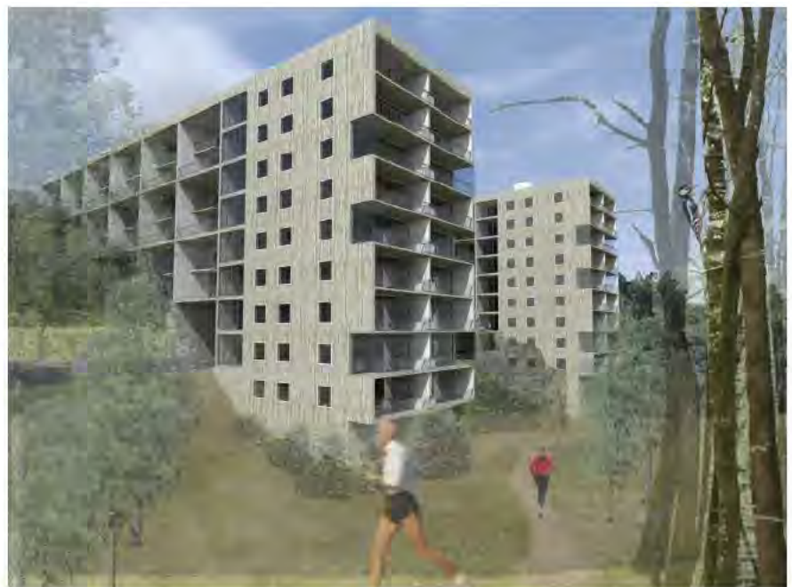
View to the North towards the middle house. The wooden facade is noticed as well as the glazed areas that get sun protection from the large terraces.
