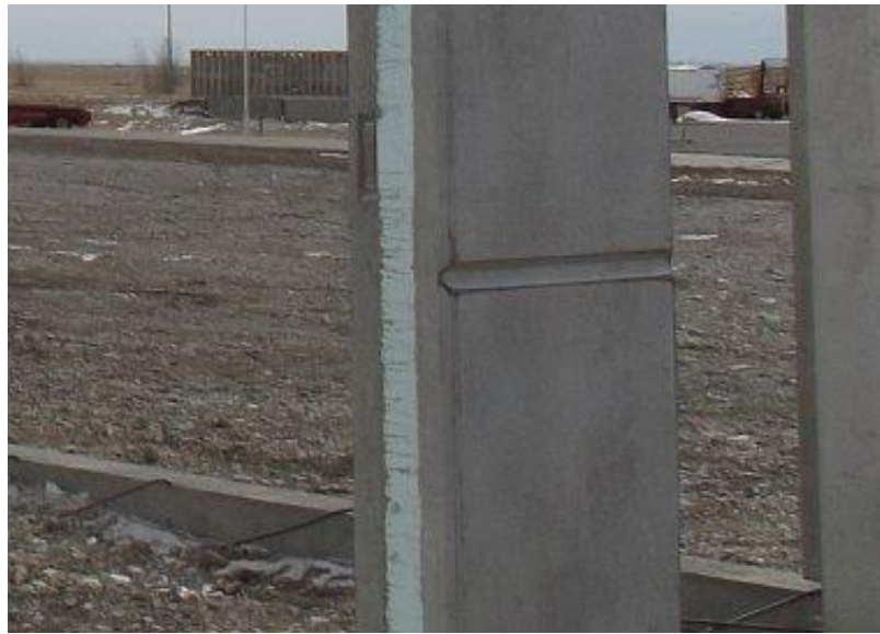
Figure 2-1 Sandwich panel, two concrete wythes parted by an insulation layer (Mountain view – pre-cast concrete©, 2015).
