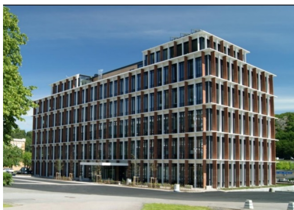
Bengt Dahlgren's Office building in Mölndal (Jönsson & Olsson, 2013).
