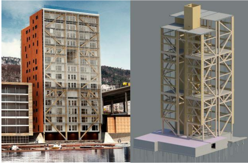
Figure 5 Model of the timber building Treet in Bergen, Norway. (Abrahamsen & Malo, 2014).
