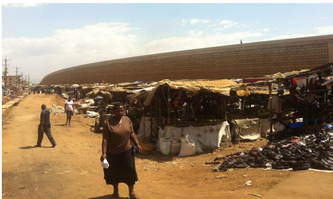
Figure 27. Kondele Market with the newly constructed wall-like flyover bypass highway in the background.
