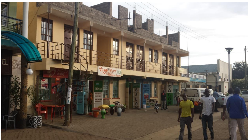
Figure 45. Example of building design with external access balconies. The photo shows an existing building in Kondele, Kisumu.
