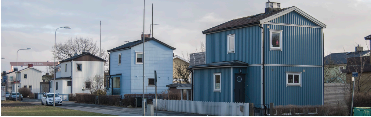
figure 35. Houses on Sommersgatan
