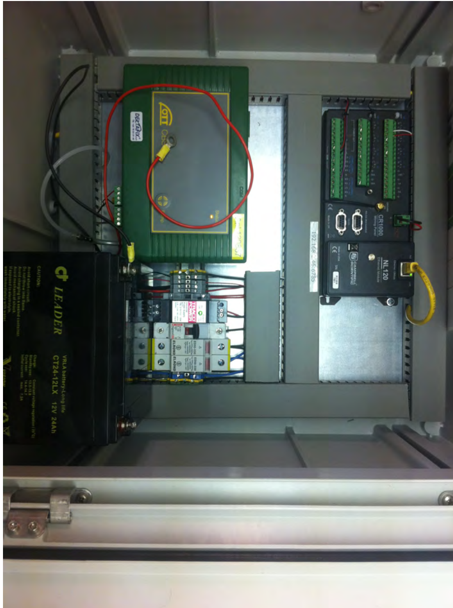
Figure 4.3: The green bubbler unit with the surrounding electronics
