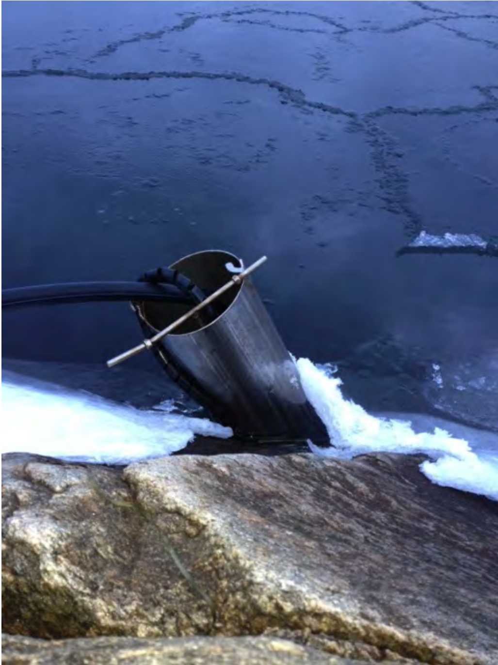
Figure 1.5: Drift ice damaging the pressure sensor casing.
