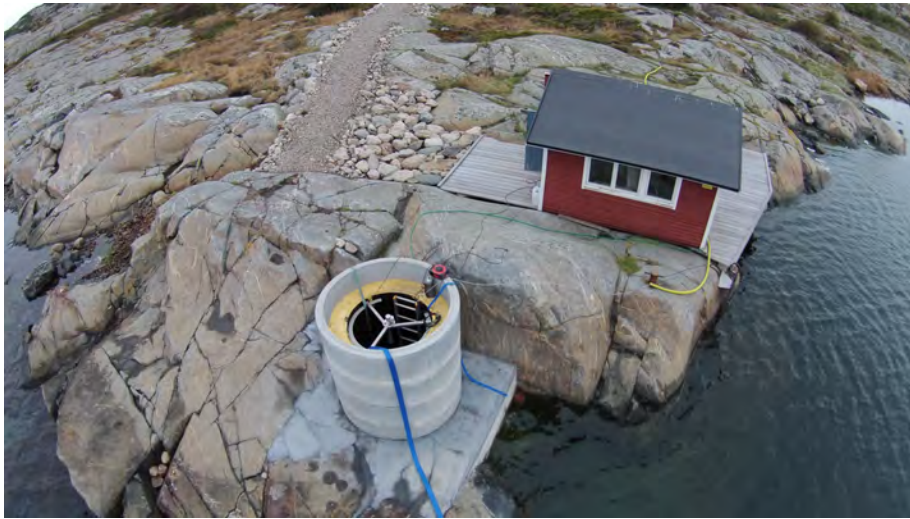
Figure 5.1: The new measurement well and the measurement hut before the installation of the sensors.
