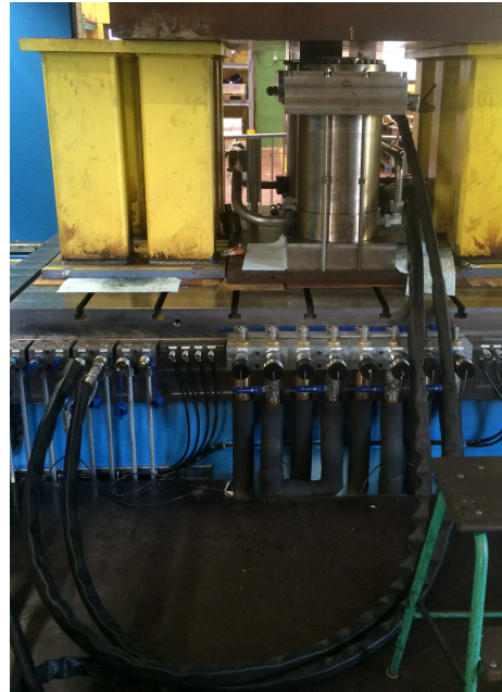
Figure 2.1: Picture of the hydraulic outlet connected to the hydraulic cylinder.
