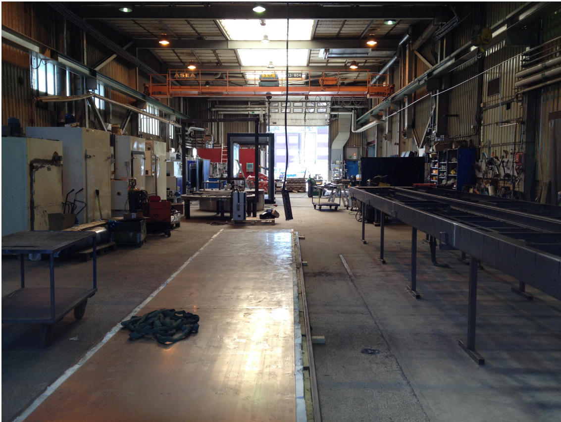
Figure 4.3: Photo of the oven building area.
