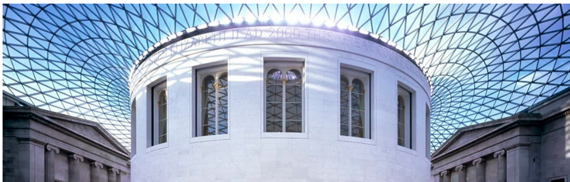
Figure 2: The roof over the British Museum Great Court designed by Foster+Partners. The form is mathematically generated by Chris Williams, but the triangularization of the grid has been form found, see [2].
