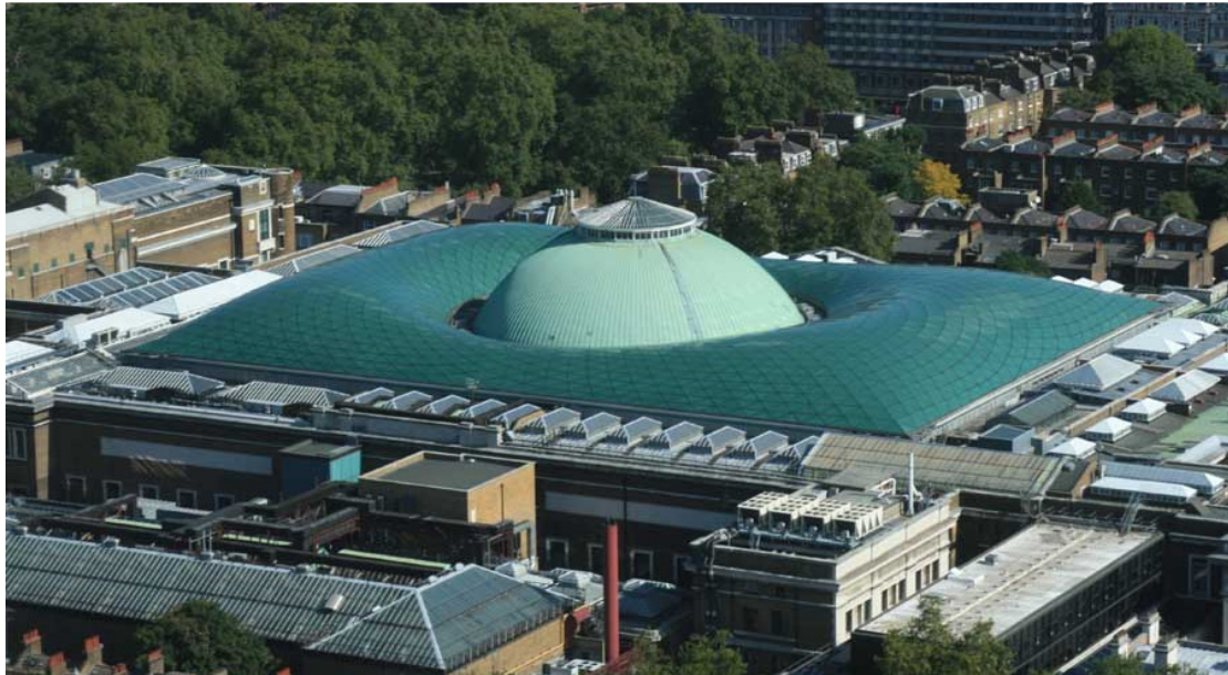
Figure 42: The roof over the Great Court from above, see [5]. A view from inside is seen on Figure 2.
