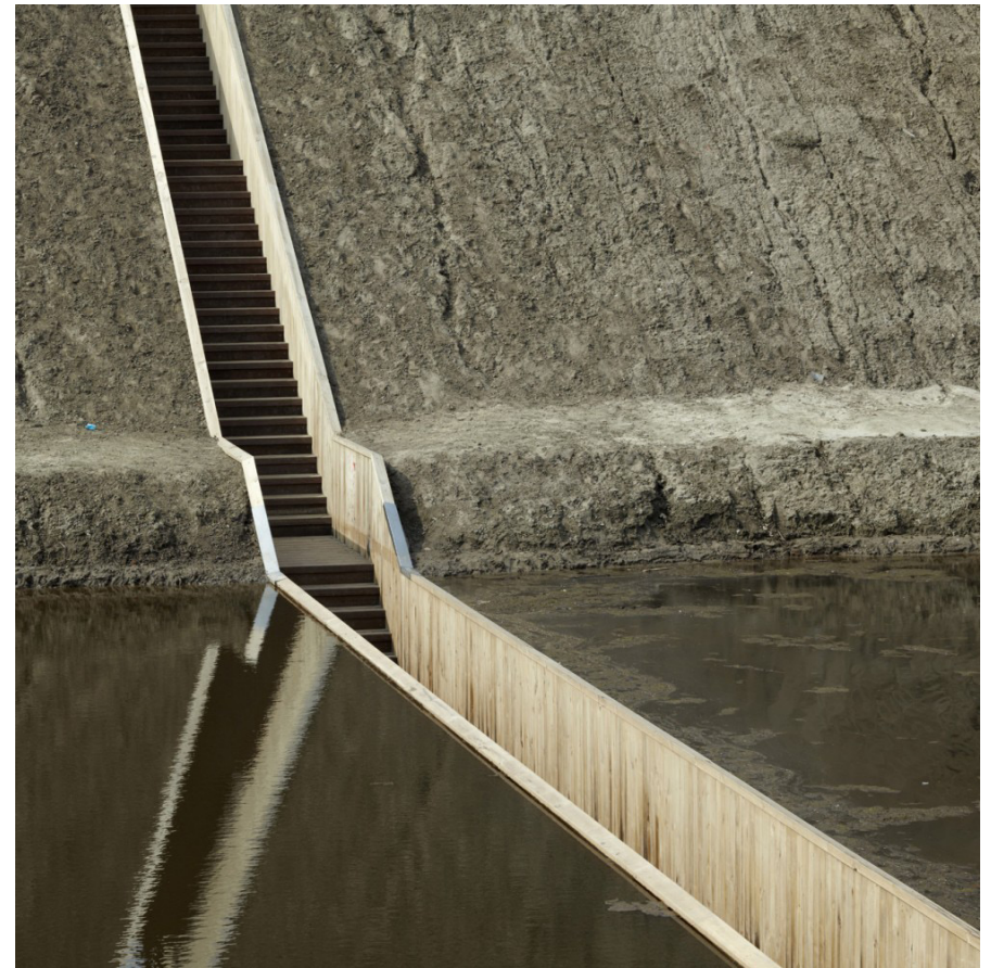
Figure 25: Picture of the Moses bridge [14].
