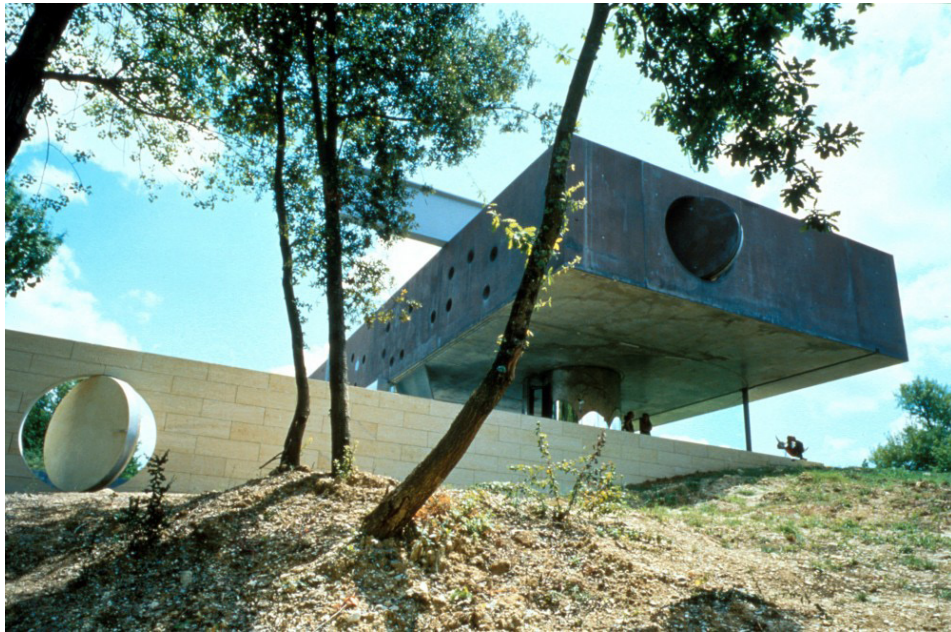
Figure 26: Picture of Maison Bordeaux [13].
