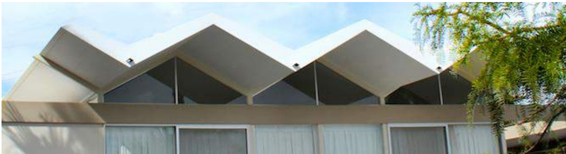
Figure 2.9 Folded steel roof in Palm Springs by Donald Wexler, built in 1962 ( Ultra Modern Style ).
