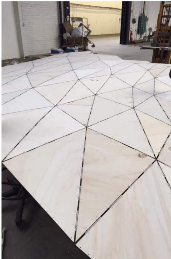
Figure 4.55 Assembling and folding of full scale structure.
