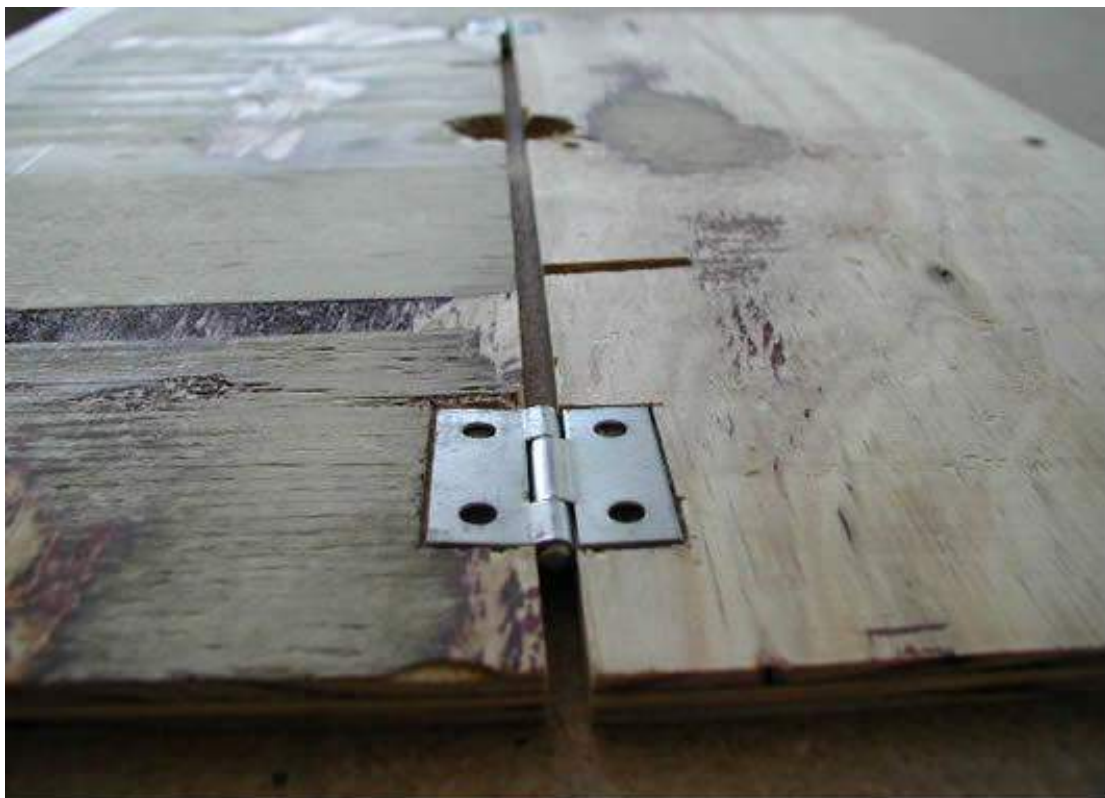
Figure 4.15 Metal hinge connection.
