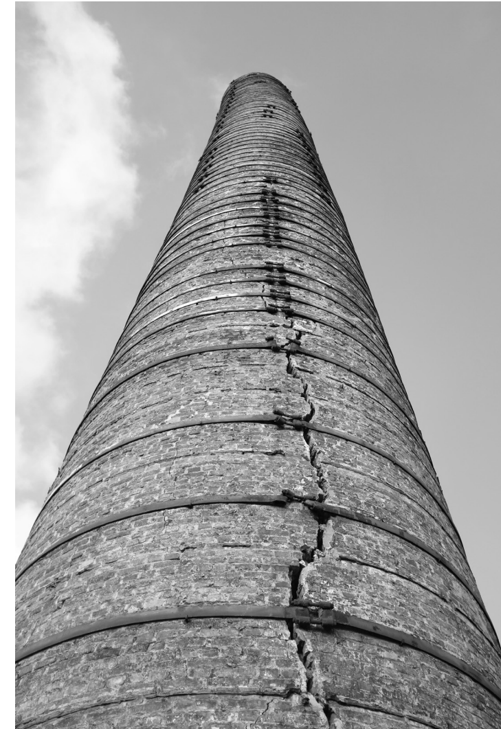
Fig. 11: Chimney Novobric - Lauwers Factory
