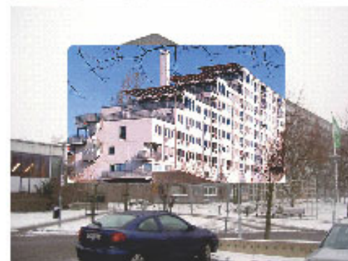
Image 9. A million programme block in Gårdsten and a montage showing its retrofitting.
