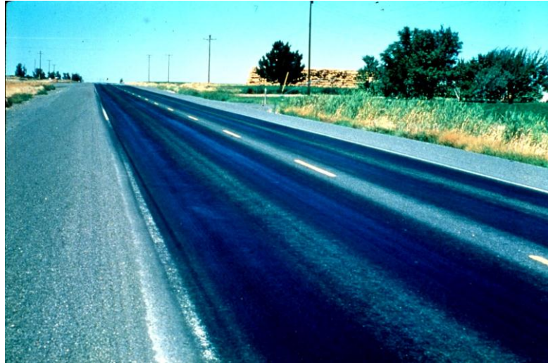
Figure 12: Bleeding in the wheel paths (Pavement Interactive, 2010)
