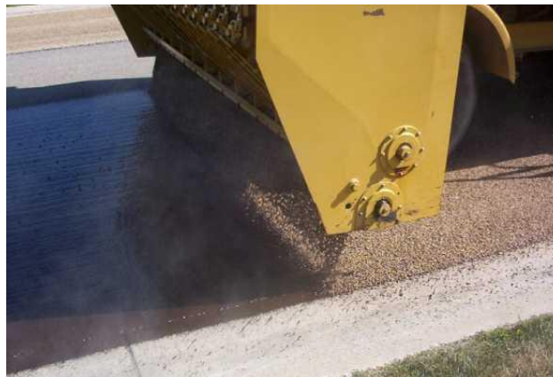
Figure 4: Chip seal coating. Spreading out aggregates on hot asphalt- rubber liquid (City of Mankano, n.d)
