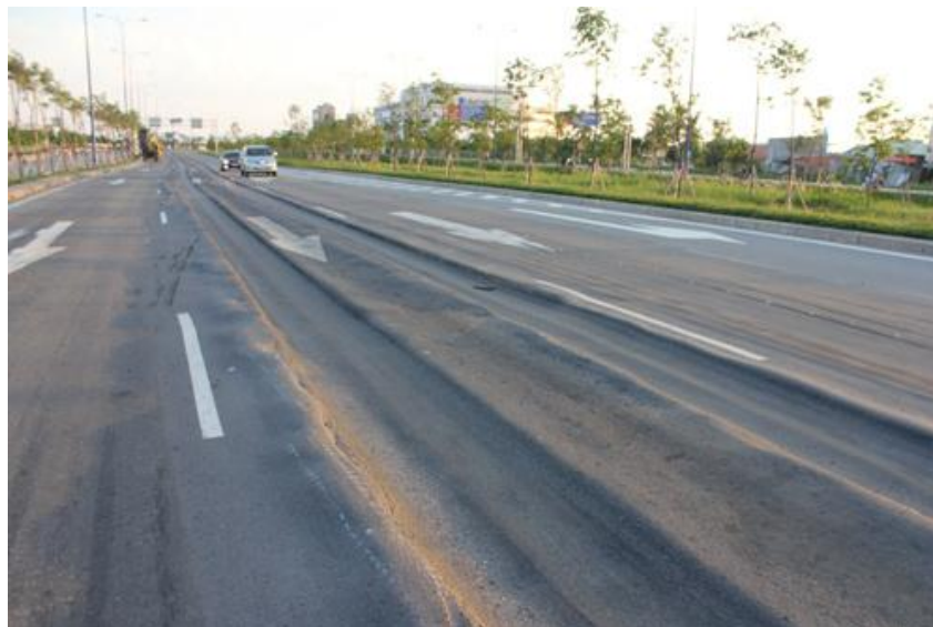
Figure 10: Extreme rutting in wheel paths (Auto Vina, 2012)
