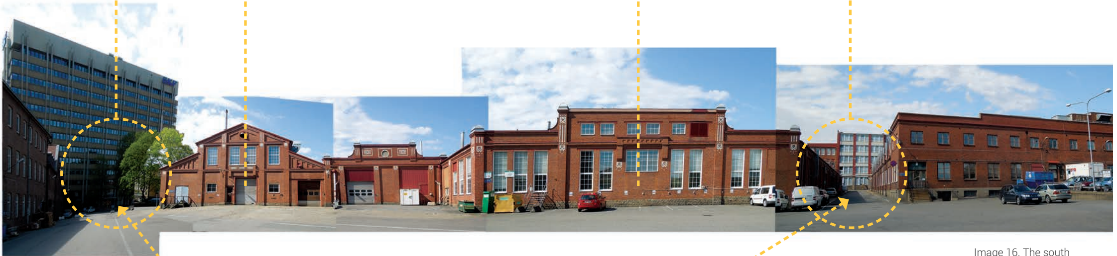
Image 16. The south facade of M-verkstaden
