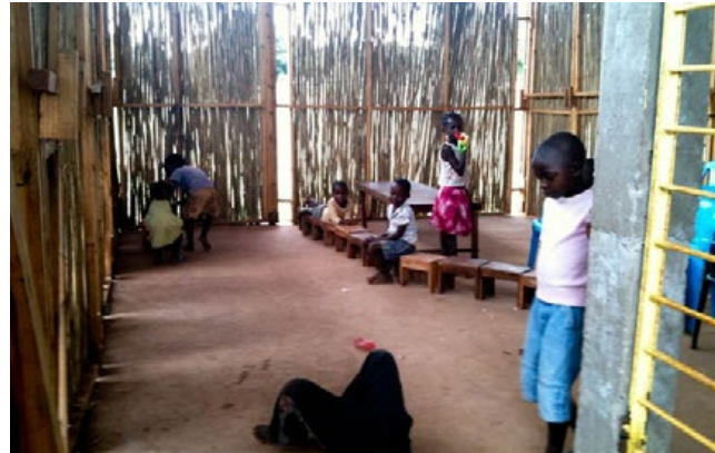
fig. 63 Stabilized soil floor
