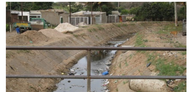
Fig.44 Clogged run-off drainage
