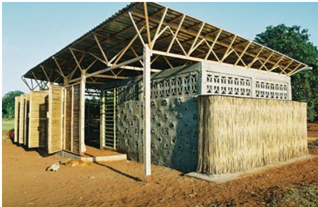
Fig.87 School in Chimundo with earthbag walls, glass bottle walls, bamboo screen doors and metal roof structure By Bergen School of Architecture (2009)
