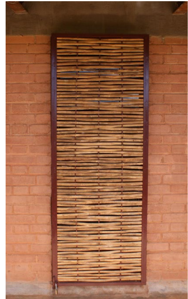
Fig.89 Manica Football for Hope Center, with Bamboo screens as shading mechanism
