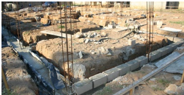
fig. 57 Concrete block foundation
