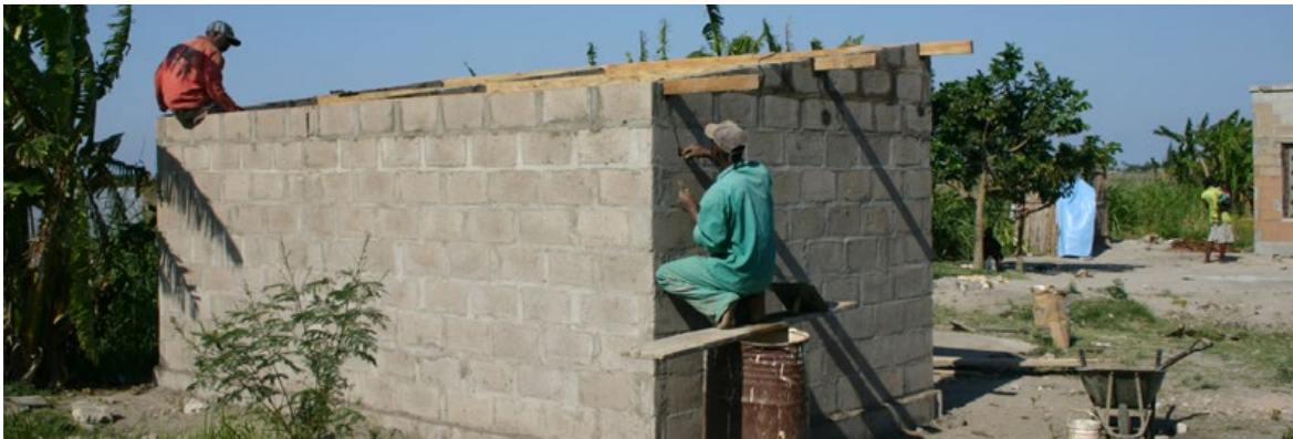
fig. 45 Virtually all residential projects are done by informally trained local builders Photo by Mauro Paul
