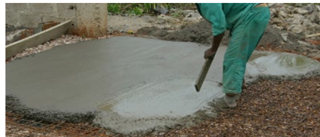
fig. 53 Reinforced concrete mixture
