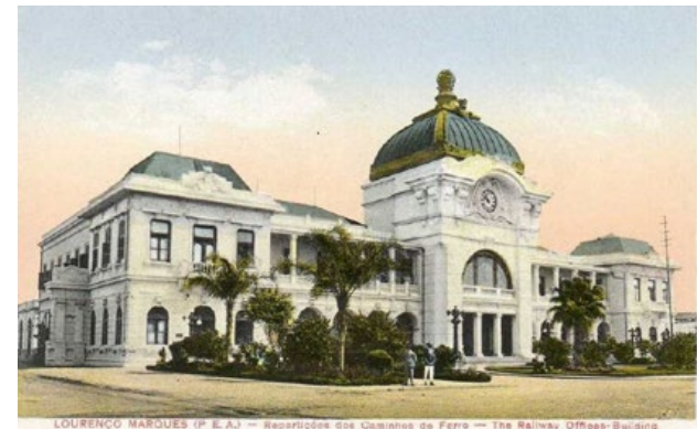
Fig.27 Railway station, built 1916
