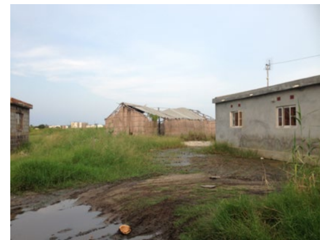
Fig.86 Soil erosion and still waters
