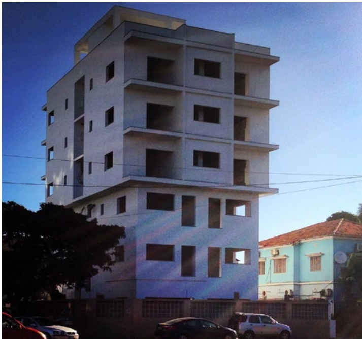
Fig.9 Two-storey house to six-storey apartment building conversion, central Maputo
