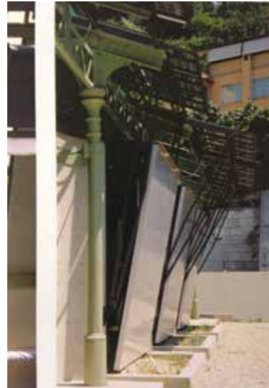
Children's Museum, Rome, Italy, with a PV system integrated into the sun protection: Abbate & Vigeveno Architectura, Rome, Italy
