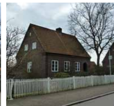
Fig. 21. Pitched roof with dark brick facade.
