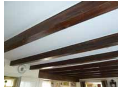
Fig.14. Visible wooden beams
