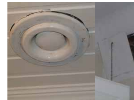
Fig. 31-32. Exhaust air and natural ventilation
