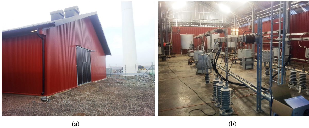
Fig. 6.38 Back-to-back HVDC Station in Gothenburg. Plot (a): collector-VSC station. Plot (b): coupling inductor and AC filters.
