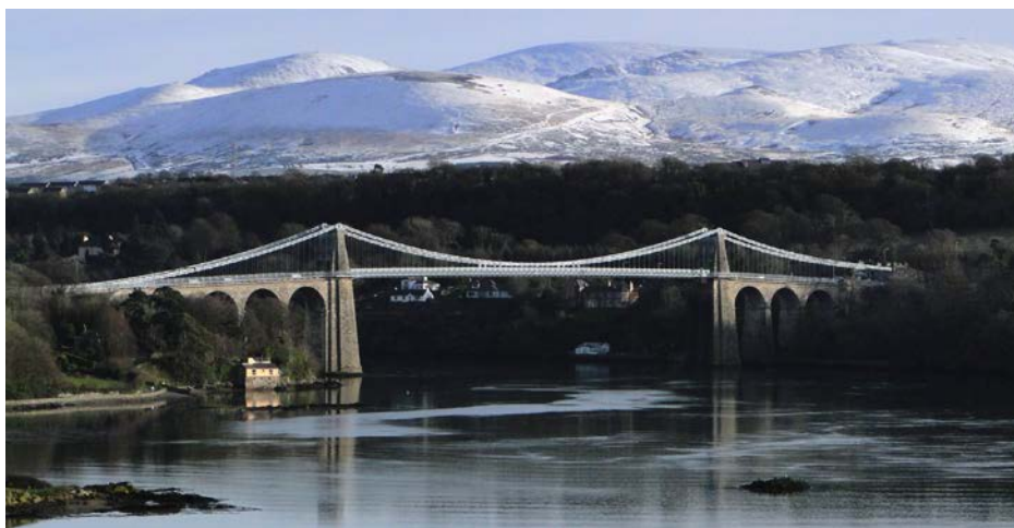
Figur 11 - Menai Suspension Bridge (1826), Wales (Knapton 2004)
