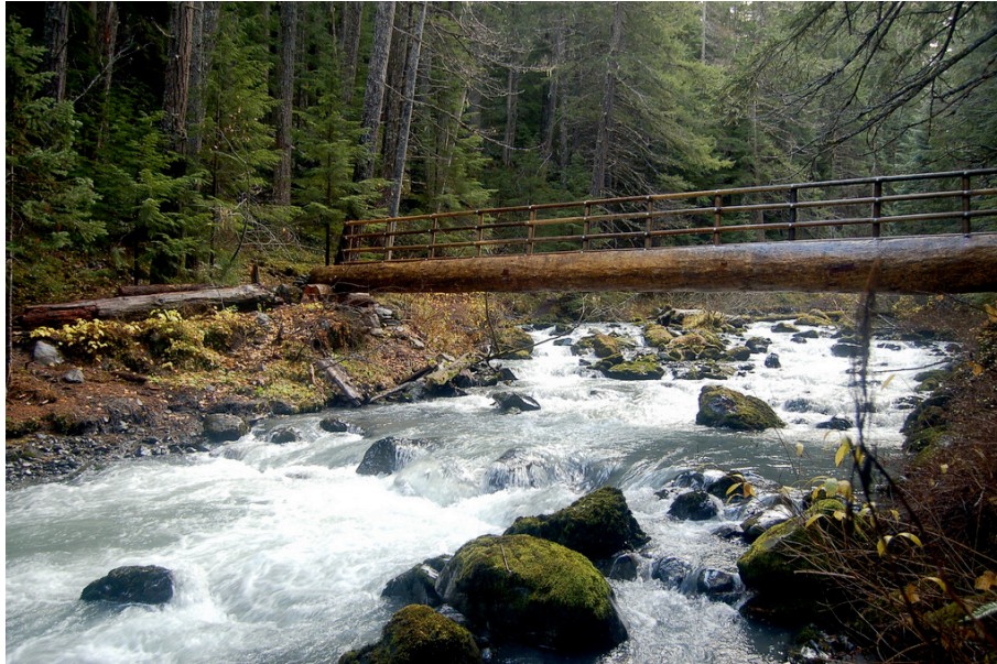
Figur 2 – Neat Log Bridge on Upper Dungeness Trail (Peterson, 2009)
