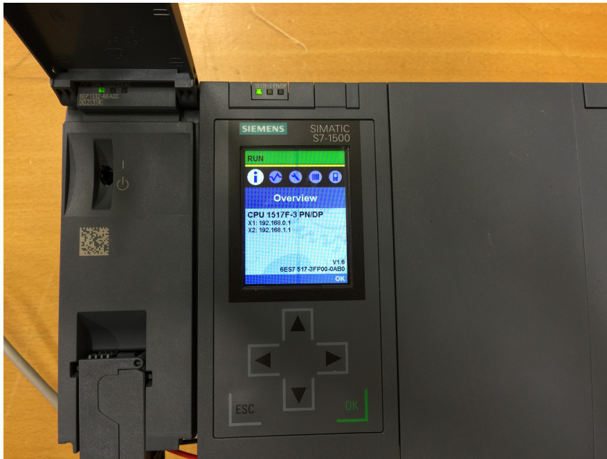
Figure 14: Powering on the PLC
