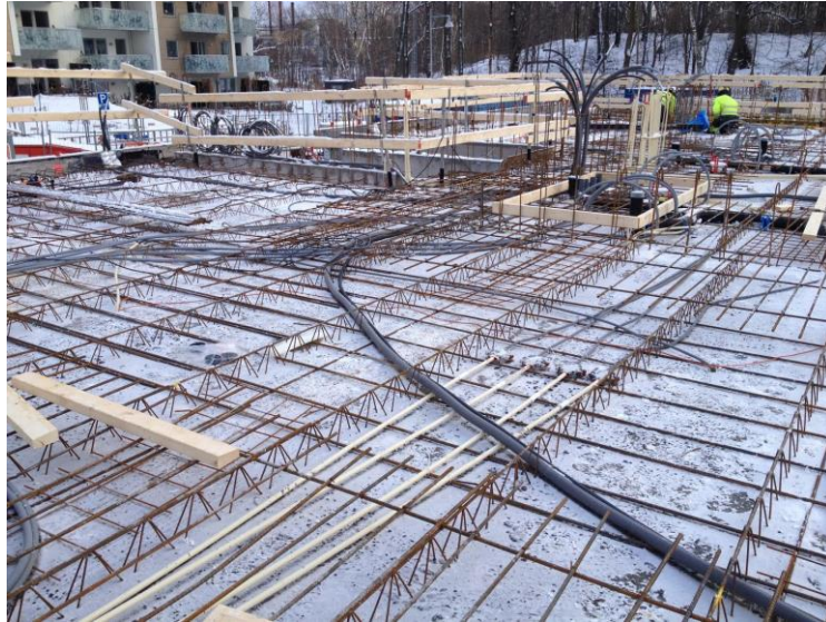
Figure 7 - Lower layer of floor reinforcement installed at a JM construction site
