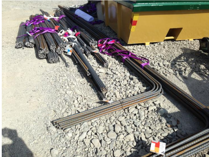
Figure 13 - Temporary storage area at the construction site
