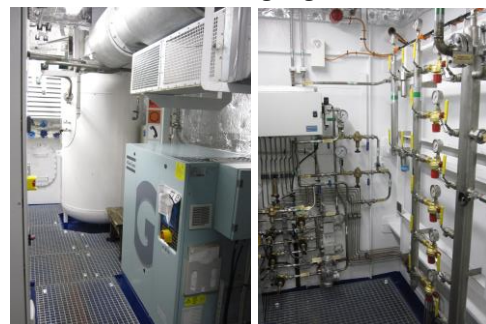
Inert gas generator room
