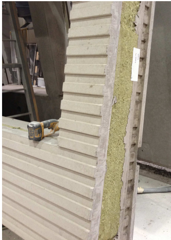
Figure 2.1 Typical construction of a sandwich element. Prefabricated wall element in the factory of the concrete supplier AB Strängbetong. (Photo: Angela Sasic Kalagasidis).
