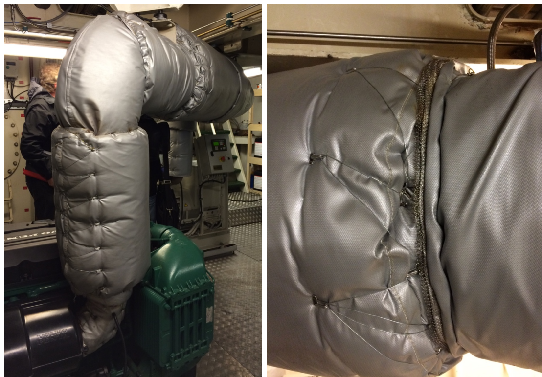
Figure 4-7 Insulation of exhaust system in cargo ferry Ärlan
