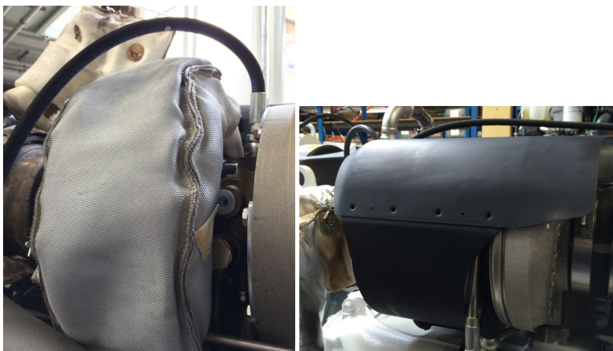
Figure 4-13 Turbocharger insulation by insulation fabric protected by a metallic cover
