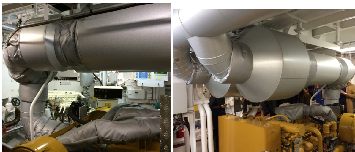
Figure 4-8 Insulation of exhaust system in cargo ferry Göta II
