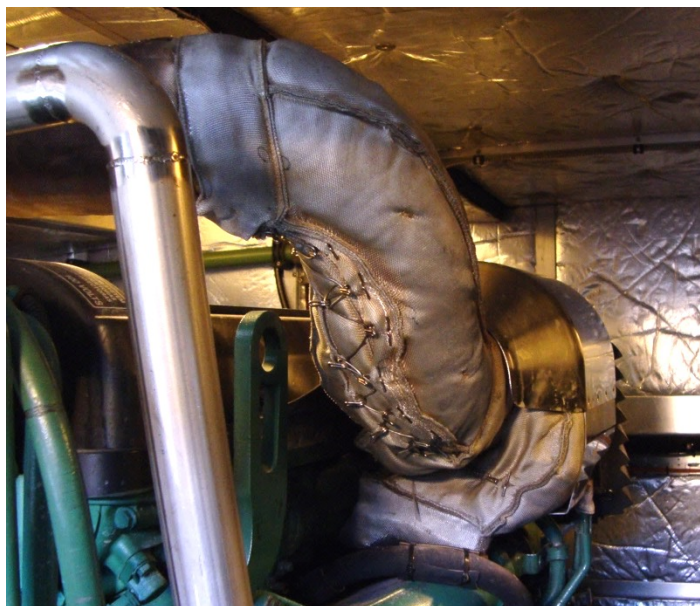
Figure 4-12 Fabric/blanket insulation of a Riser
