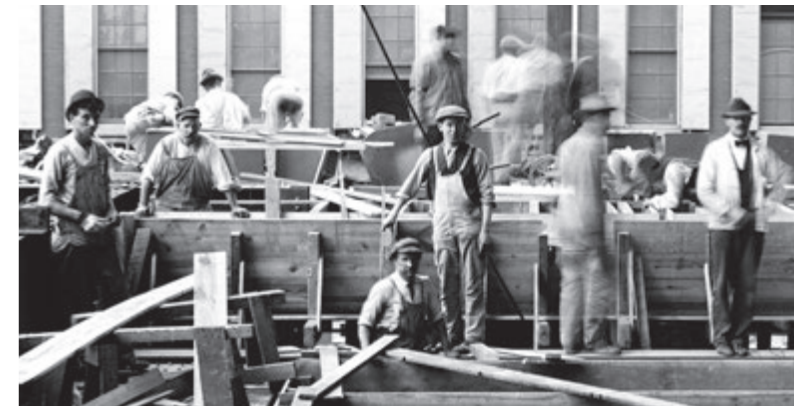
Picture 27. Carpenters and Masons, Frankford EL Construction in 1913. The building in the back was established in 1868.
