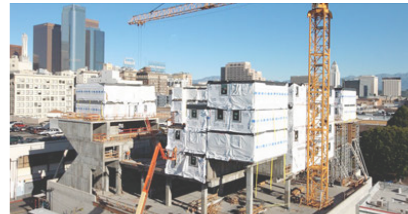
Picture 28. How a construction site can appear today. This is "Star Apartments" in Los Angeles, 2013.
