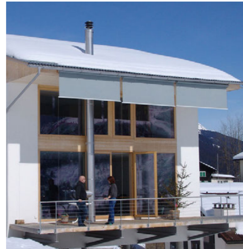
Picture 19. The Strohhaus Braun-Dubuis by Werner Schmidt, situated in the Swiss Alps, is a load-bearing construction with jumbo bales that are 1,2 meters wide (Minke and Mahlke, 2005).
