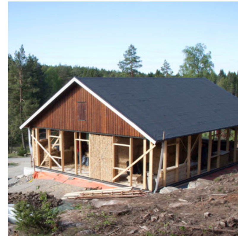
Picture 20. Infill straw bale construction in the spring of 2014. The house at Korpaberget in Alingsås, Sweden.
