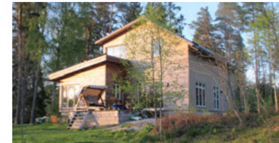
Picture 22. The house of Ingrid Faldner with both plaster and wood siding. With wood paneling on the most weather-exposed side of the house.
