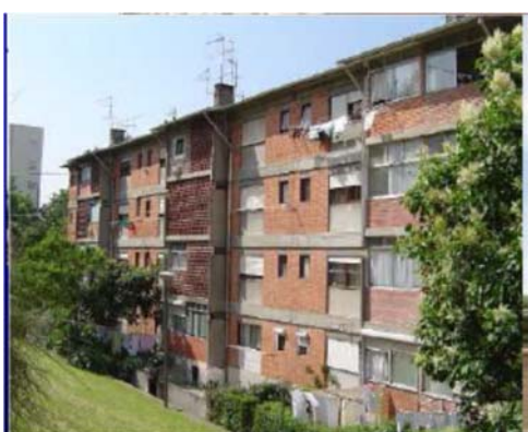
Damaged brick veneer of the cavity wall. Inner wall is of concrete.
