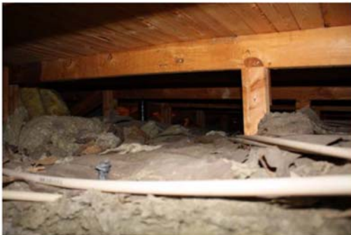
The status of the ventilated cold attic before the retrofitting
