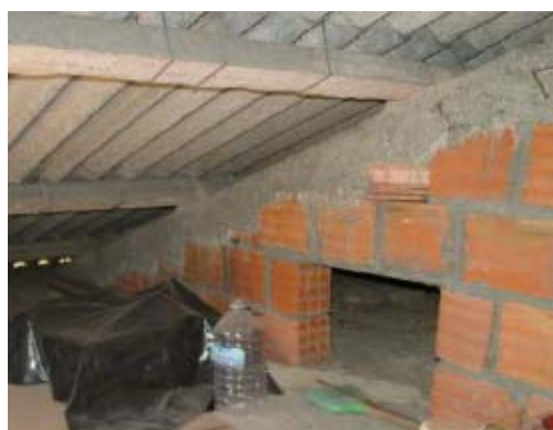
Mould on the wall in the kitchen.
