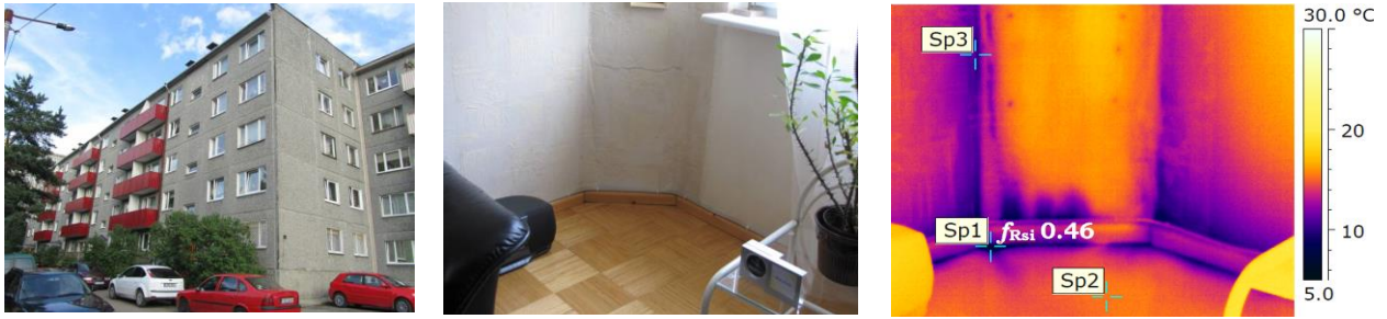
Figure 12. External view of the case study building before the renovation (left) and junction of external walls at inserted ceiling of a cellar as a regular photo (middle) and a thermal image (right).
