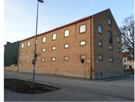
3. Existing warehouse. This building is currently being rebuilt into apartments and will have a light coloured plastered facade after the refurbishment.
