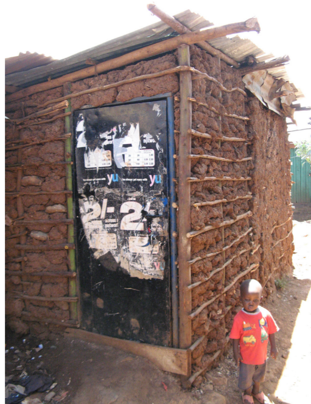
Current site view 4
