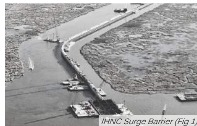
IHNC Surge Barrier (Fig 1)
