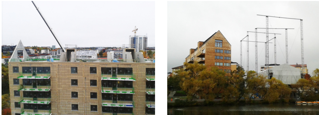
Figure 24. House A in construction without protection. House C next to B raised with height-adjustable tent.
