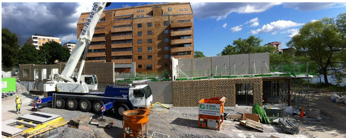
Figure 16. Construction of House A in prefab concrete twin walls and plate slabs (Boetten, 2013).
