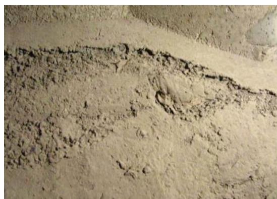
*Figure 34 Voids and pits on concrete is found in the inclined web at L-23#.*
