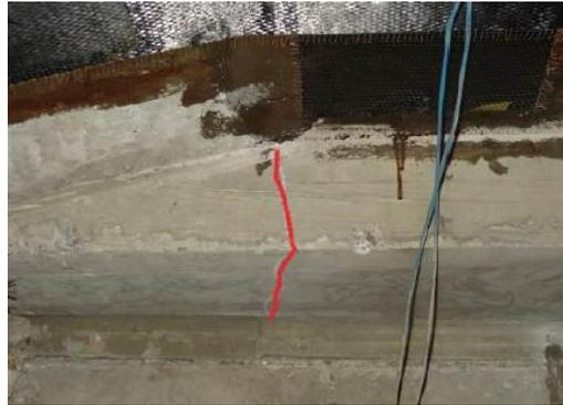
Figure 28 L-shaped crack is found in the roof of some testing chambers.
