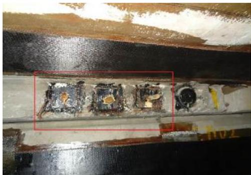
Figure 31 Rusting of anchor head is found at the toothed plate at L-29#.
