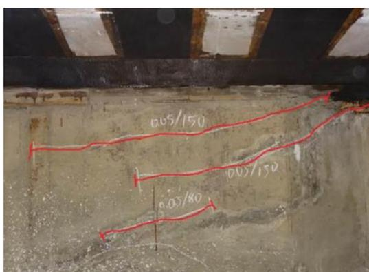
*Figure 33 Diagonal crack is found in the inclined web at L-19#.*
