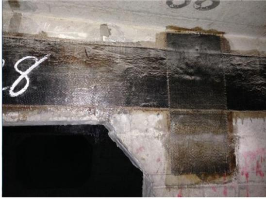
Figure 11 In 2008, CFRP was pasted to the roof and diaphragm in order to control cracks.
