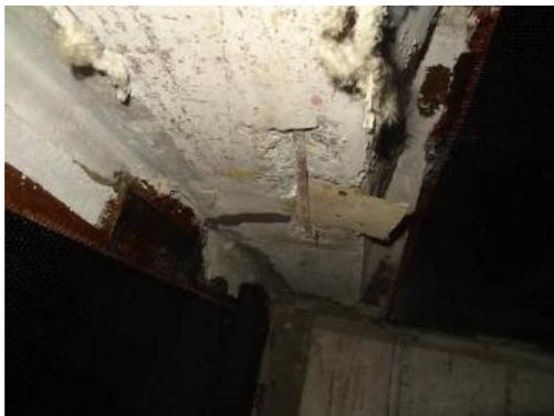
Figure 29 Exposure of reinforcement is found in the toothed plate at L-52#.
