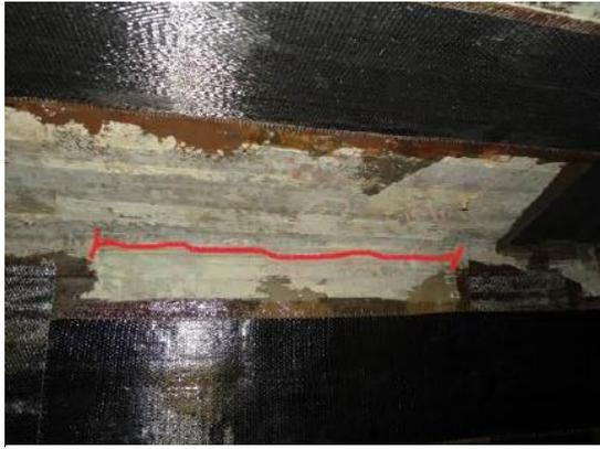
Figure 36 Transverse crack is found in the diaphragm at L-34#.
