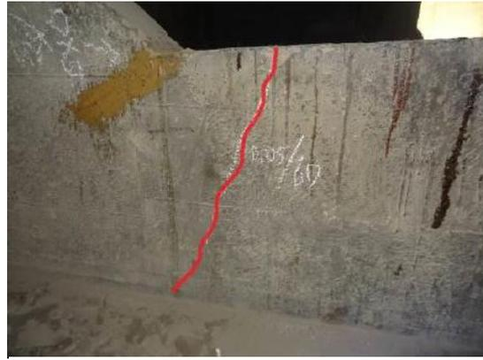
Figure 37 Diagonal crack is found in the diaphragm at L-12#.
