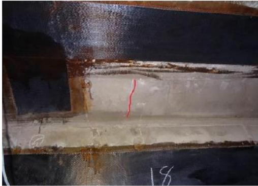
Figure 27 Longitudinal crack is found in the roof of some testing chambers.
