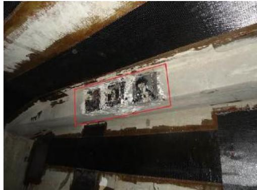
Figure 30 Seepage and bleaching is found in anchor head at the toothed plate in L-22#.
