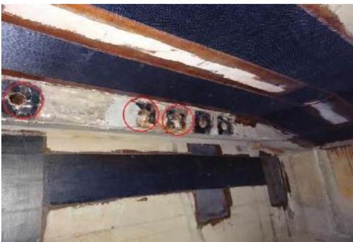
Figure 32 Rusting of reserved prestressing pipe is found in the toothed plate at R-29#.
