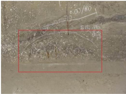
Figure 35 Exposure of reinforcement is found in the inclined web at L-17#.
