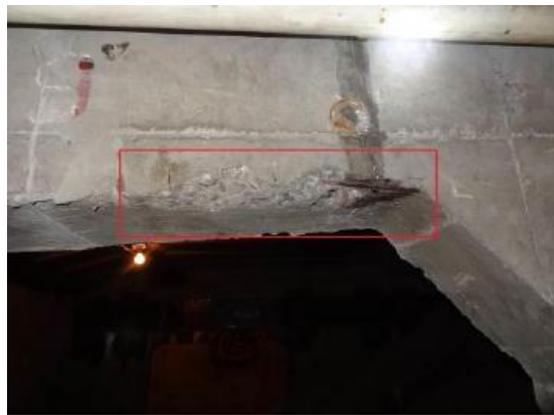
Figure 39 Exposure of reinforcement is found in diaphragm L-19#.
