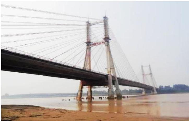
*Figure 7 Jinan Yellow River Highway Bridge is a double tower and double cable planes suspension prestressed concrete cable-stayed bridge.*
