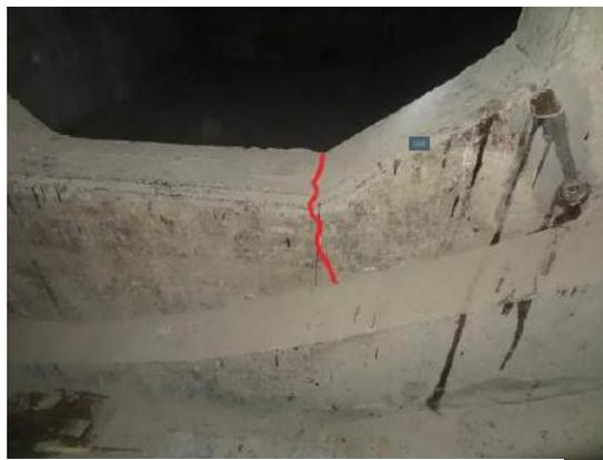
Figure 38 L-shaped crack is found in diaphragm at L-28#.
