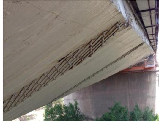
Figure 12 In 2008, steel plate was pasted to the webs.
