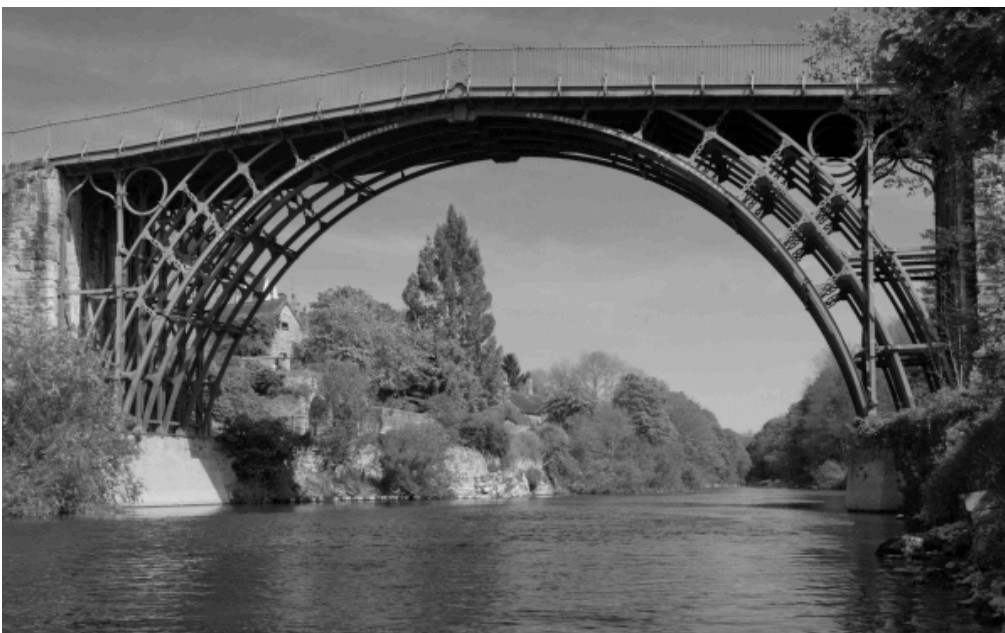
Figure 2.6 The Iron Bridge, England, the world's first cast iron bridge, design inspired wood bridge building techniques.
