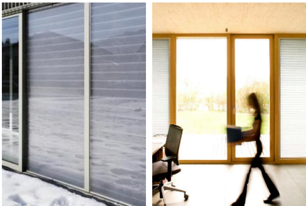
Figure 3.6 GLASSX, solar wall with PCM
