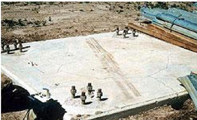
*Figure 3.8 Cracks due to temperature, Portland cement association (2005)*
