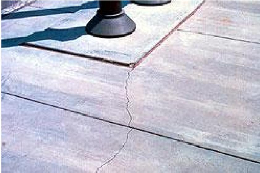
*Figure 3.6 Cracks due to drying shrinkage, Portland cement association (2005)*
