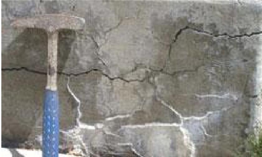
*Figure 3.10 Cracks due to Alkali-aggregate reaction, Portland cement association (2005)*
