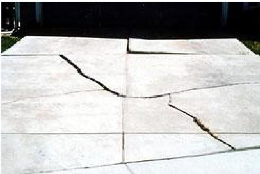
*Figure 3.11 Cracks due to Loss of support, Portland cement association (2005)*
