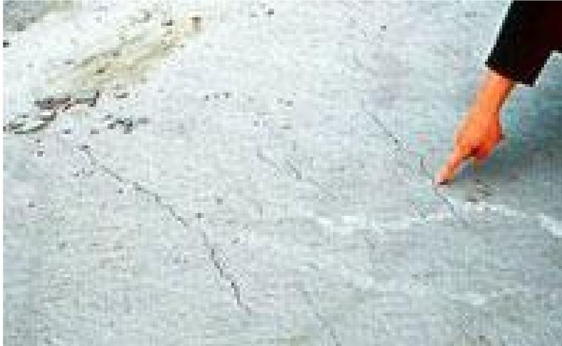
*Figure 3.7 Cracks due to plastic shrinkage, Portland cement association (2005)*
