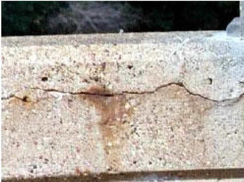
Figure 3.9 Cracks due to corrosion, Portland cement association (2005)
