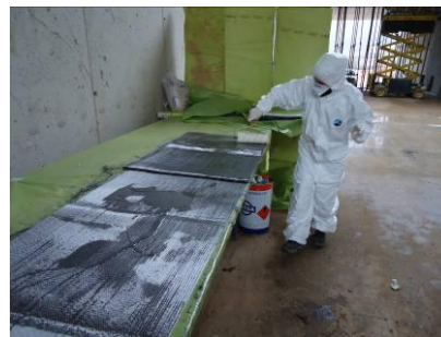
Preparation of resin for laminate impregnation
