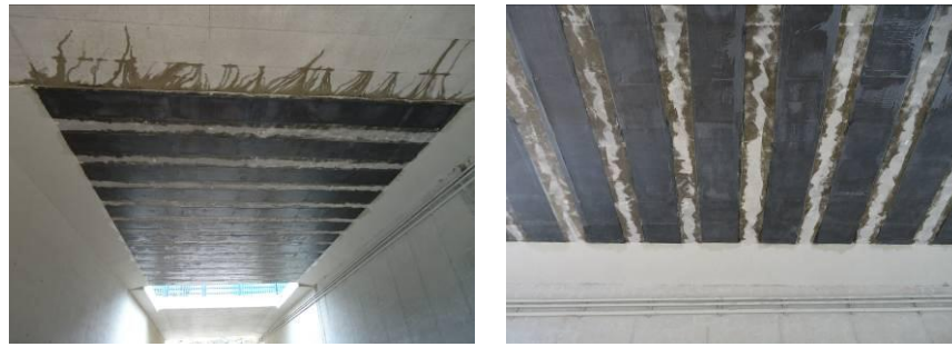
Figure 4.16 Final FRP reinforcement with carbon fiber and epoxy resin
