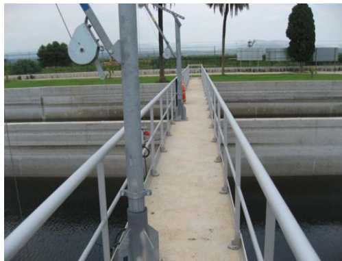
Figure 4.1 Footbridge over the biological digester
