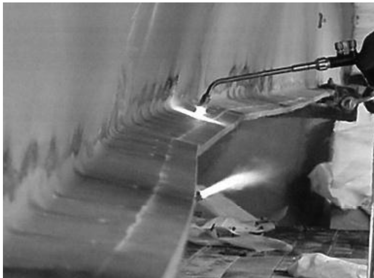
Figure 10.4 New Road Overbridge-heat straightening
