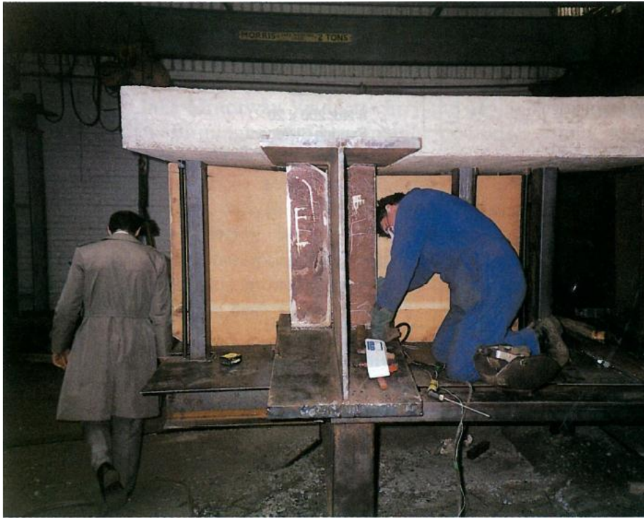
Figure 1.2 Bearing stiffener welding trial
