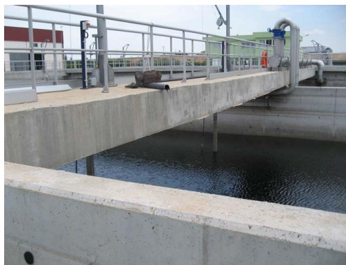
Figure 4.3 Deformations up to 4cm in the first span of one of the footbridges
