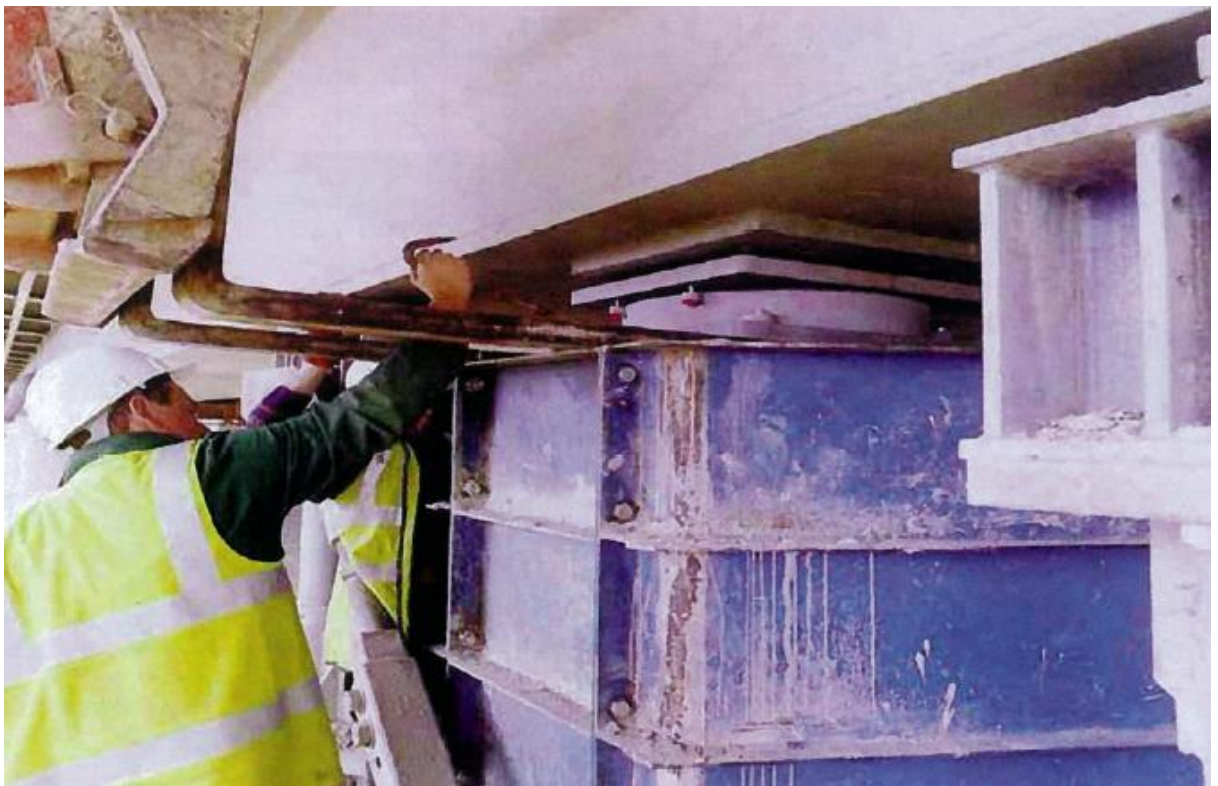
Figure 3.5 Installation of new bearing
