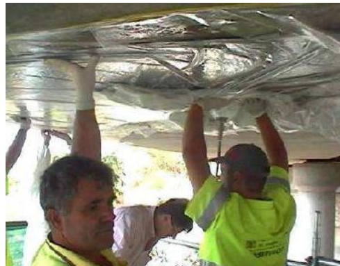
Figure 4.10 Installation of vacuum system
