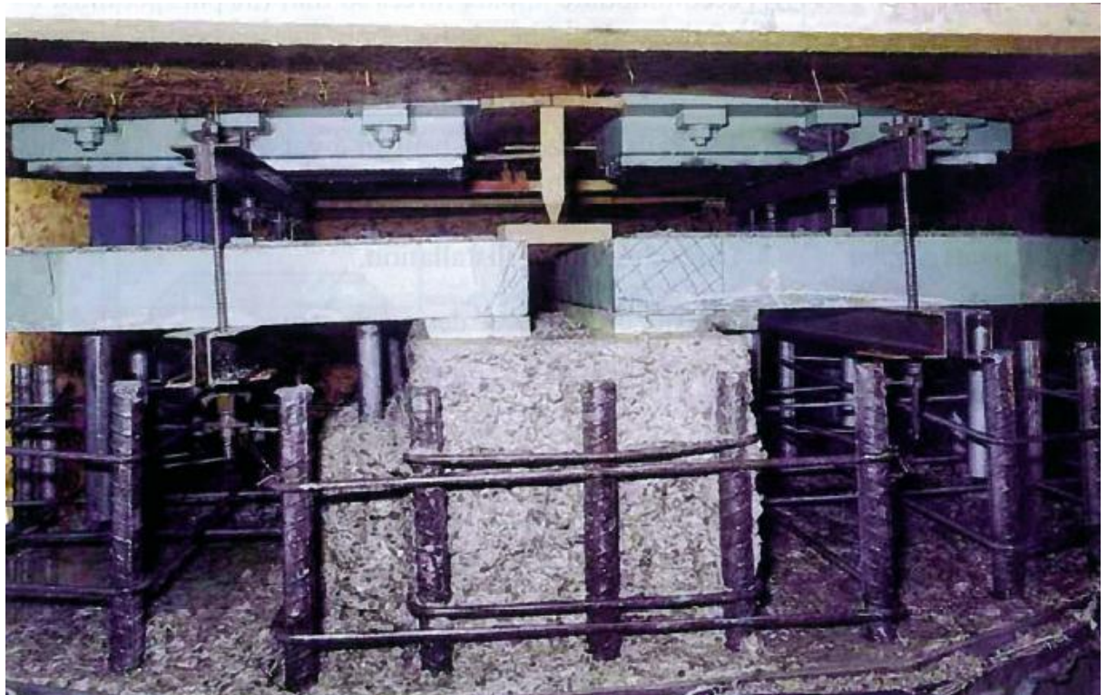
Figure 3.7 Pier top after hydrodemolition
