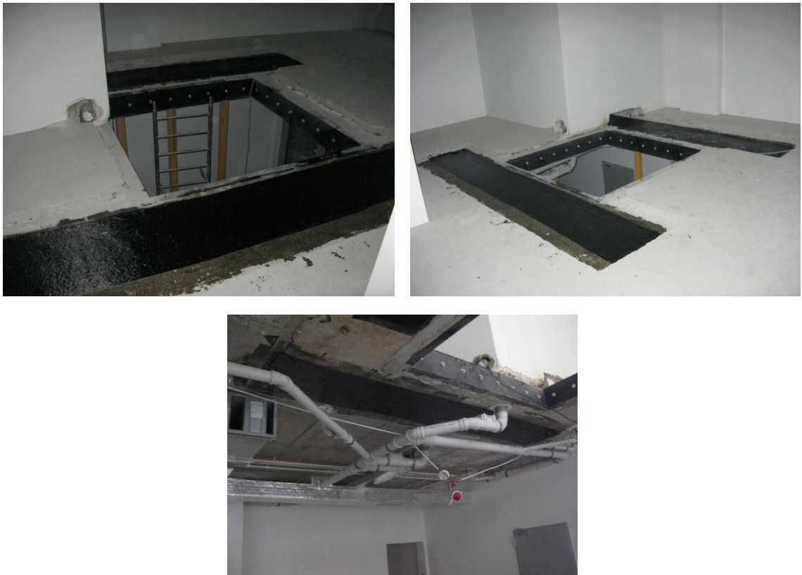
Figure 4.17 FRP reinforcement with carbon fiber and epoxy resin on the floor and opening in residential building.
