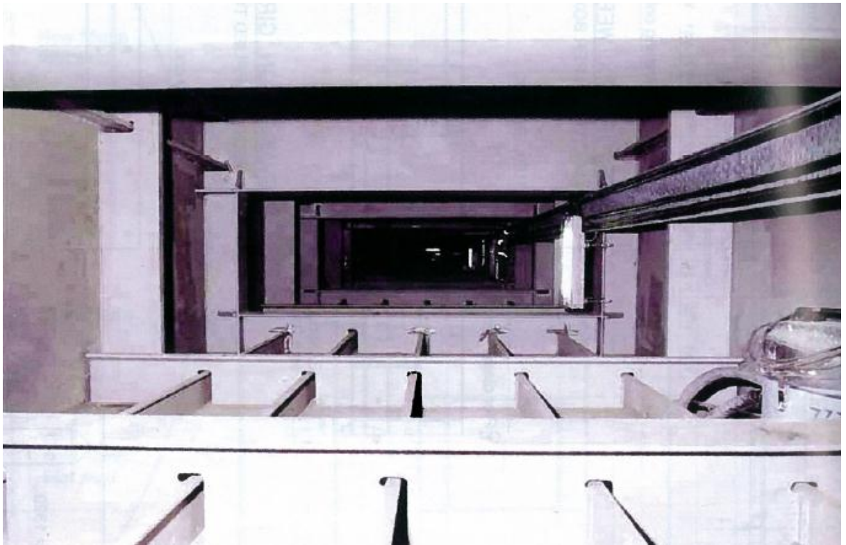
Figure 3.4 View in box showing bottom flange stiffeners
