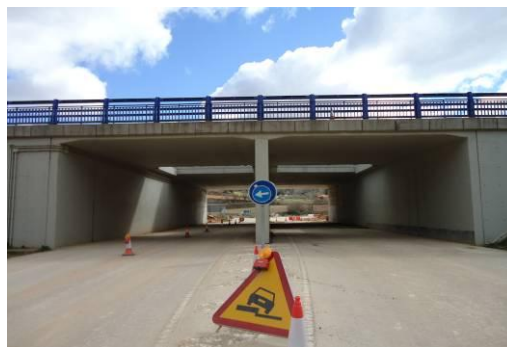
Figure 4.11 Initial situation of the project site (Motorway A-2 in Spain)
