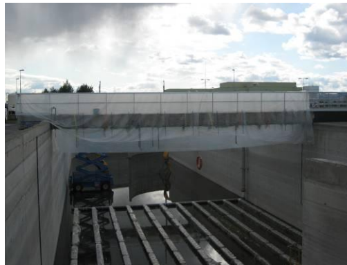
Figure 4.6 Protection of the CFRP reinforcement during curing period
