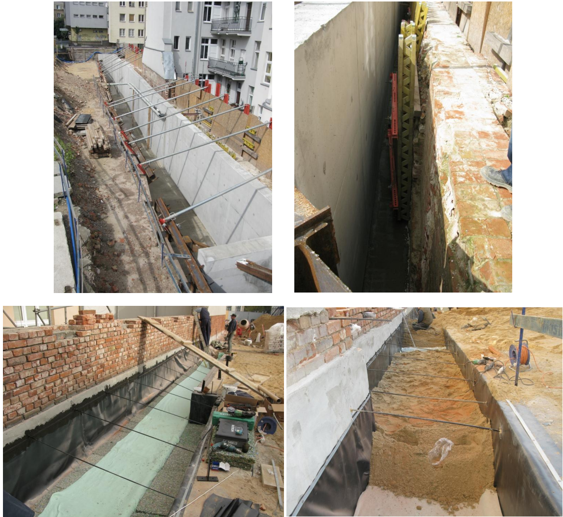
Figure 4.18 Strengthening of historical brick-wall with FRP carbon bars in Warsaw.
