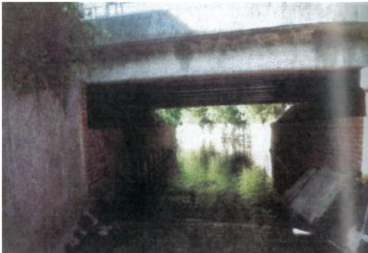
Figure 7.2 Honey Lane Bridge
