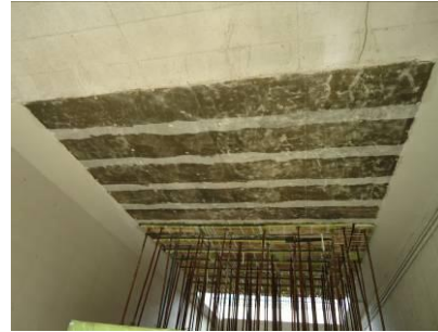
Surface preparation and impregnation
