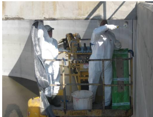
Figure 4.4 Hand-lay-up process, impregnation of fibres
