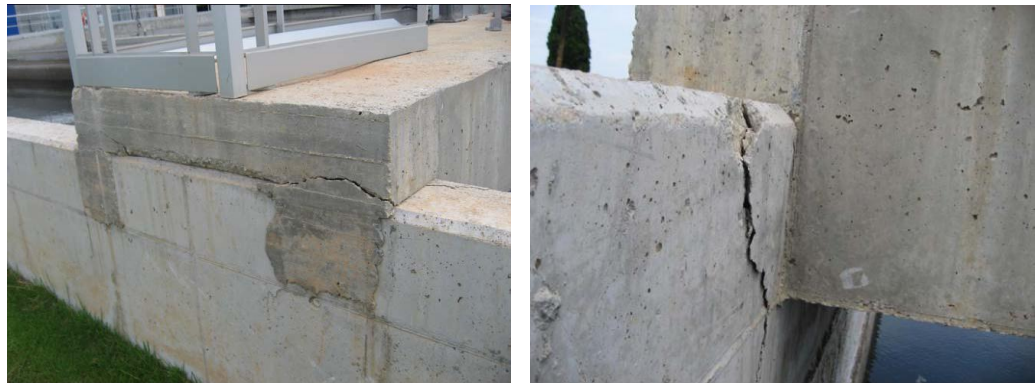
Figure 4.2 Cracks in the abutments
