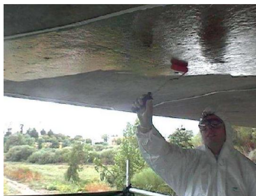
Figure 4.7 Resin impregnation of the surface
