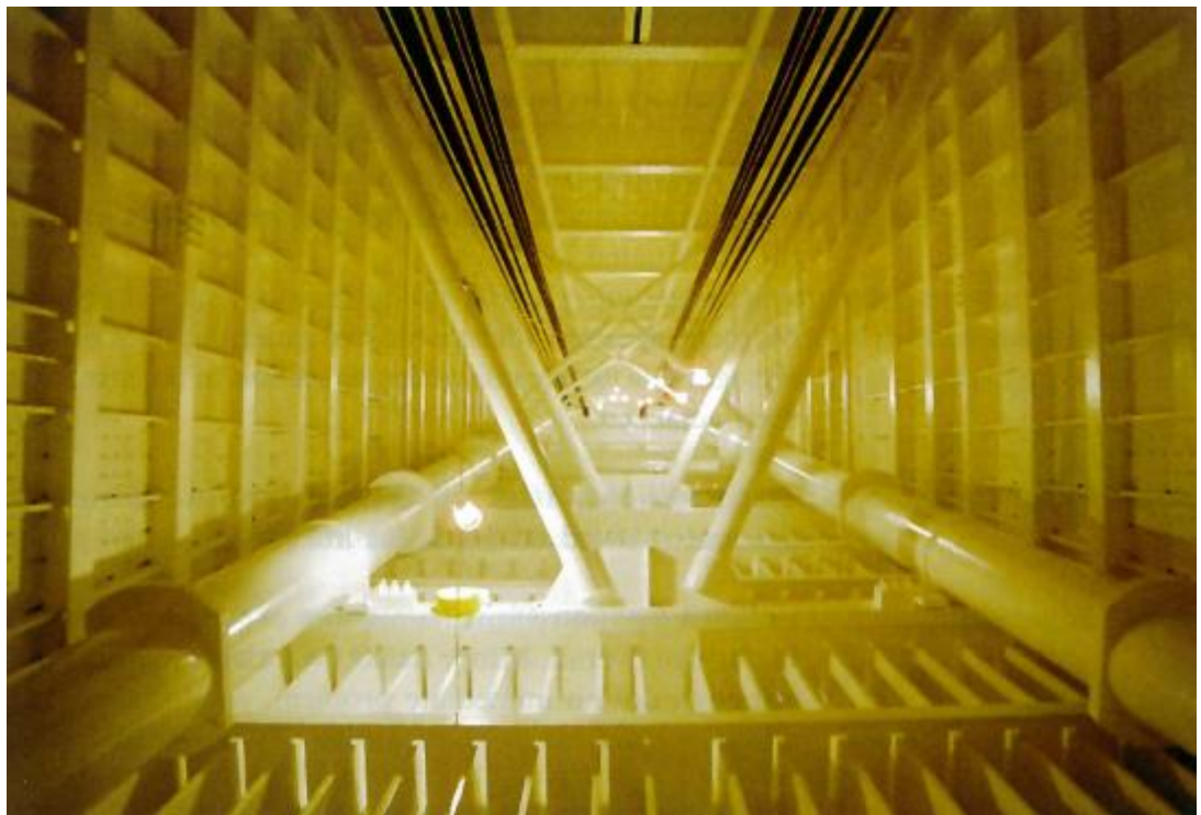
Figure 9.5 Avonmouth Bridge main span
