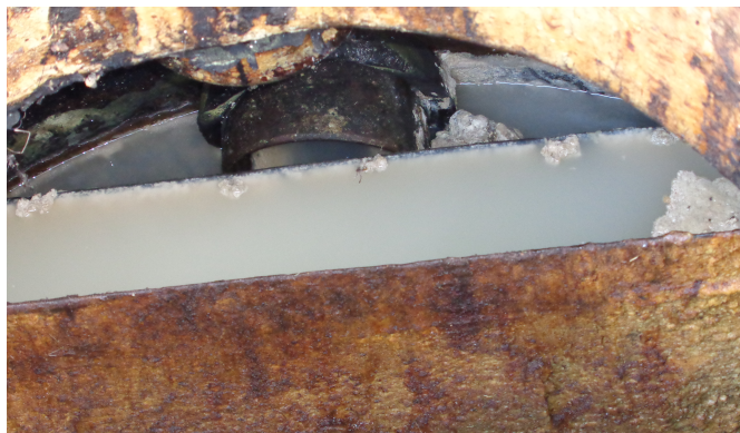
Figure 11: Fat builds up in the effluent compartment of the GS at Restaurant Syster O Bror.
