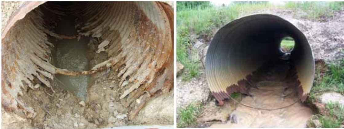
Figure 2.16 Corrugated steel culvert invert corrosion [8], [9]
