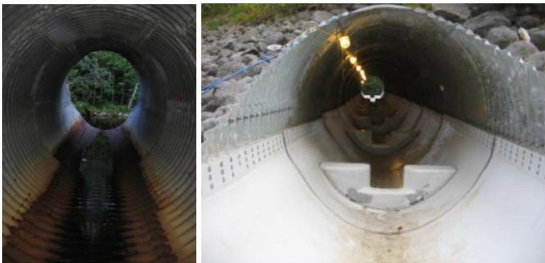
Figure 2.17 Corrosion of corrugated culvert and completed installation [10]
