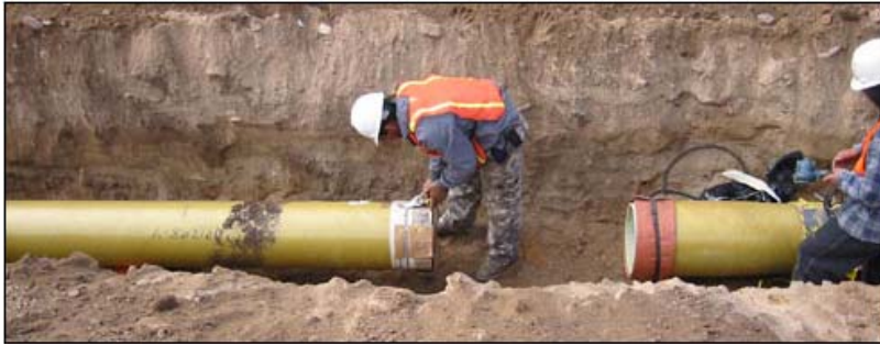
Figure 2.24 FRP underground pipe installation [17]
