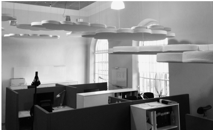
Figure 4.2.: The office after the absorbing panels and screens were installed.
