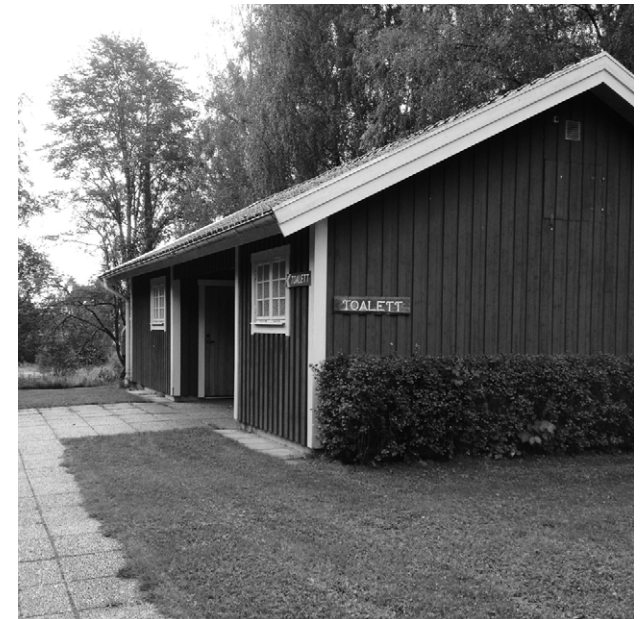
A public toilet is the first building visitors approach.
