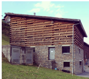
Caminada Vrin Contemporary timber structures.
