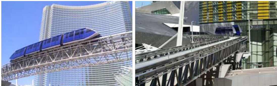
Figure 21. Tubular guideways for cable cars in Las Vegas [32].
