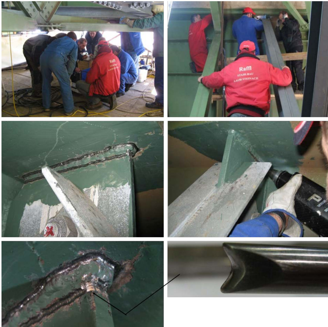
Figure 28. PIT-treated details on the Gschnitztal Bridge [38].
