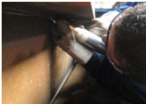
Treatment of flange/web welds
