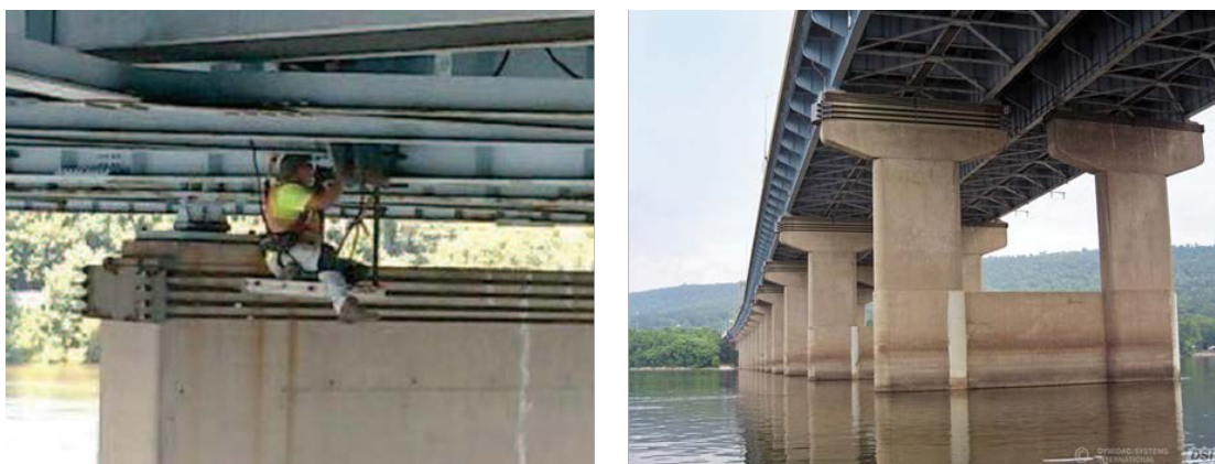
Figure 29. UIT treatment on the George N. Wade Memorial Bridge [39][40].
