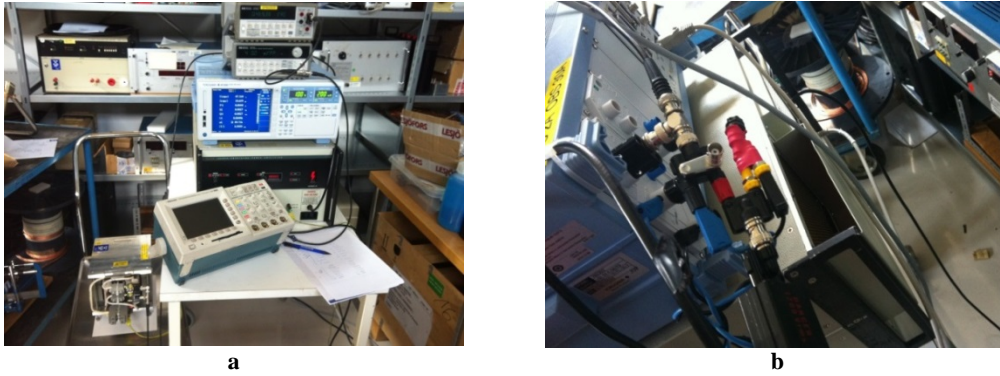
Figure 5-18: Test circuit (a) and the 2 A fast fuse in series with LV side in a red fuse holder (b).
