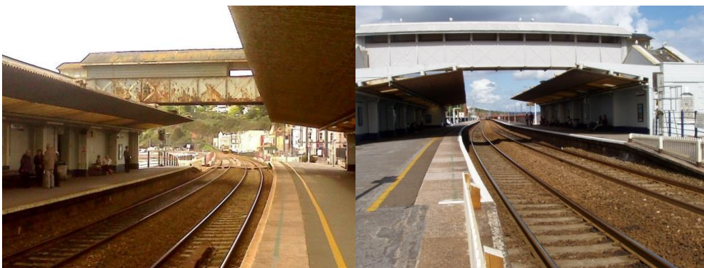
Figure 2.23 Dawlish railway station steel bridge replacement [15] with FRP composites [16]
