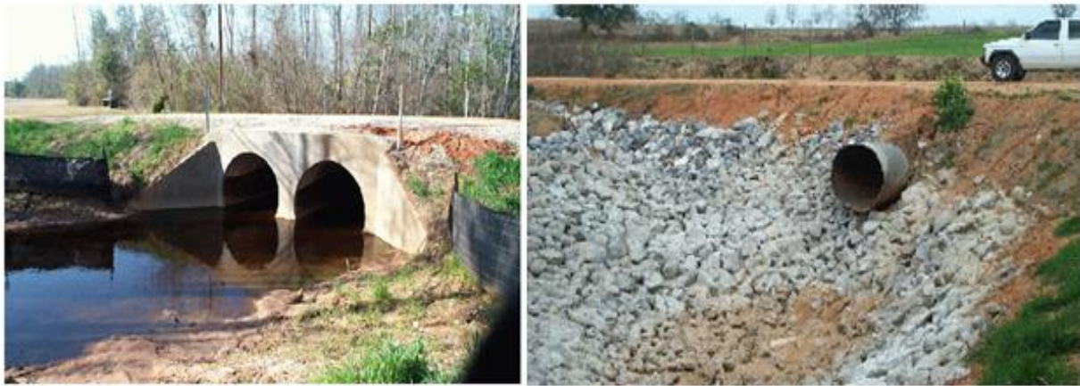
Figure 2.14 Culverts for stream crossing and drainage [6]
