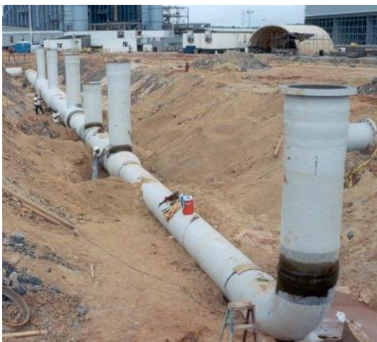
Figure 2.26 FRP water piping system at an Oregon cogenerating power facility [19]
