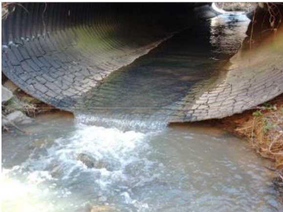
Figure 2.15 Deteriorated invert and perched end of pipe culvert [7]
