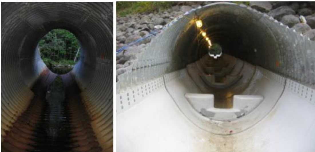
Figure 2.17 Corrosion of corrugated culvert and completed installation [10]
