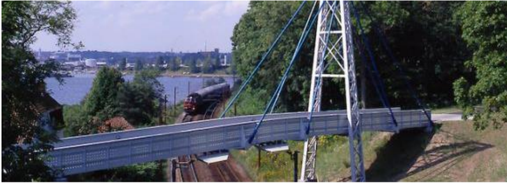
Figure 2.21 The Fiberline bridge at Kolding, Denmark [14]
