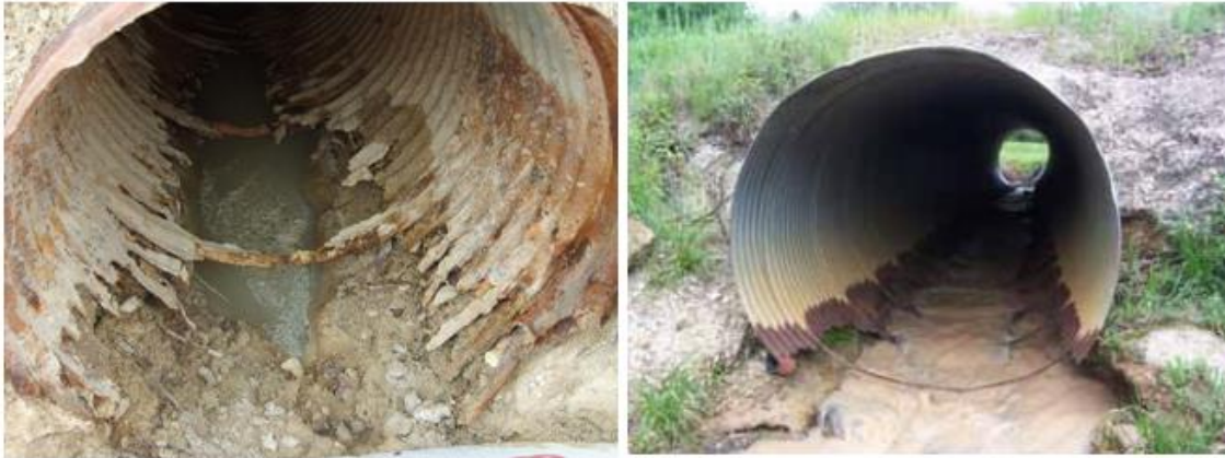
Figure 2.16 Corrugated steel culvert invert corrosion [8], [9]
