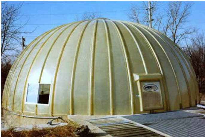
Figure 2.19 Fibreglass reinforced plastic composite digester dome [12]
