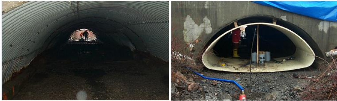
Figure 2.18 An entire culvert re-lining in Buffalo, New York, USA [11]
