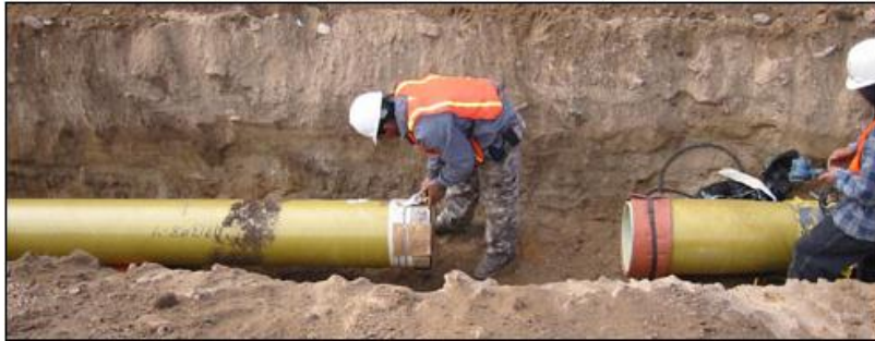
Figure 2.24 FRP underground pipe installation [17]
