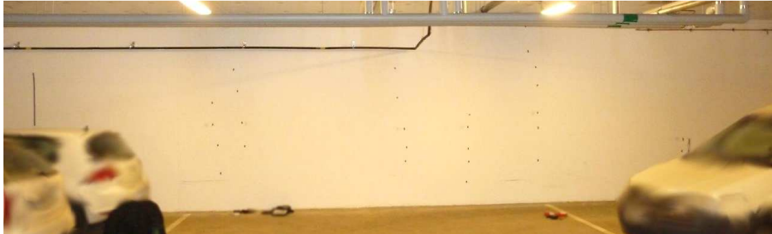
Figure 4.6 Overview of wall 1
