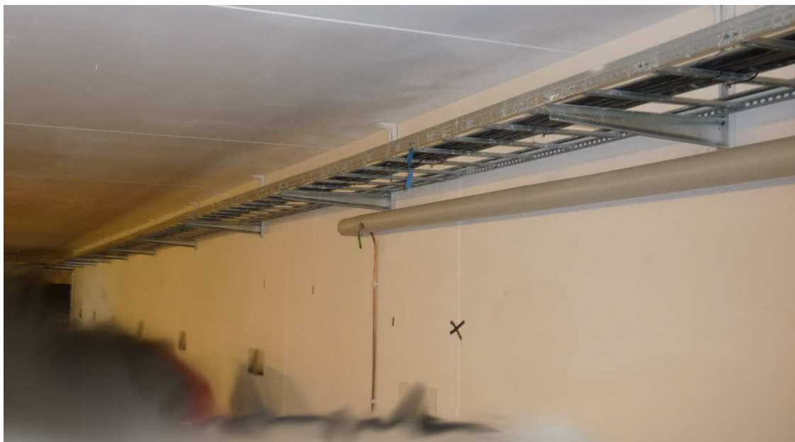
Figure 4.14 Overview of the right part of wall 2, object A
