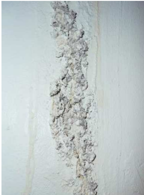
Figure 2.1 Flaking of paint near a crack due to moisture penetration
