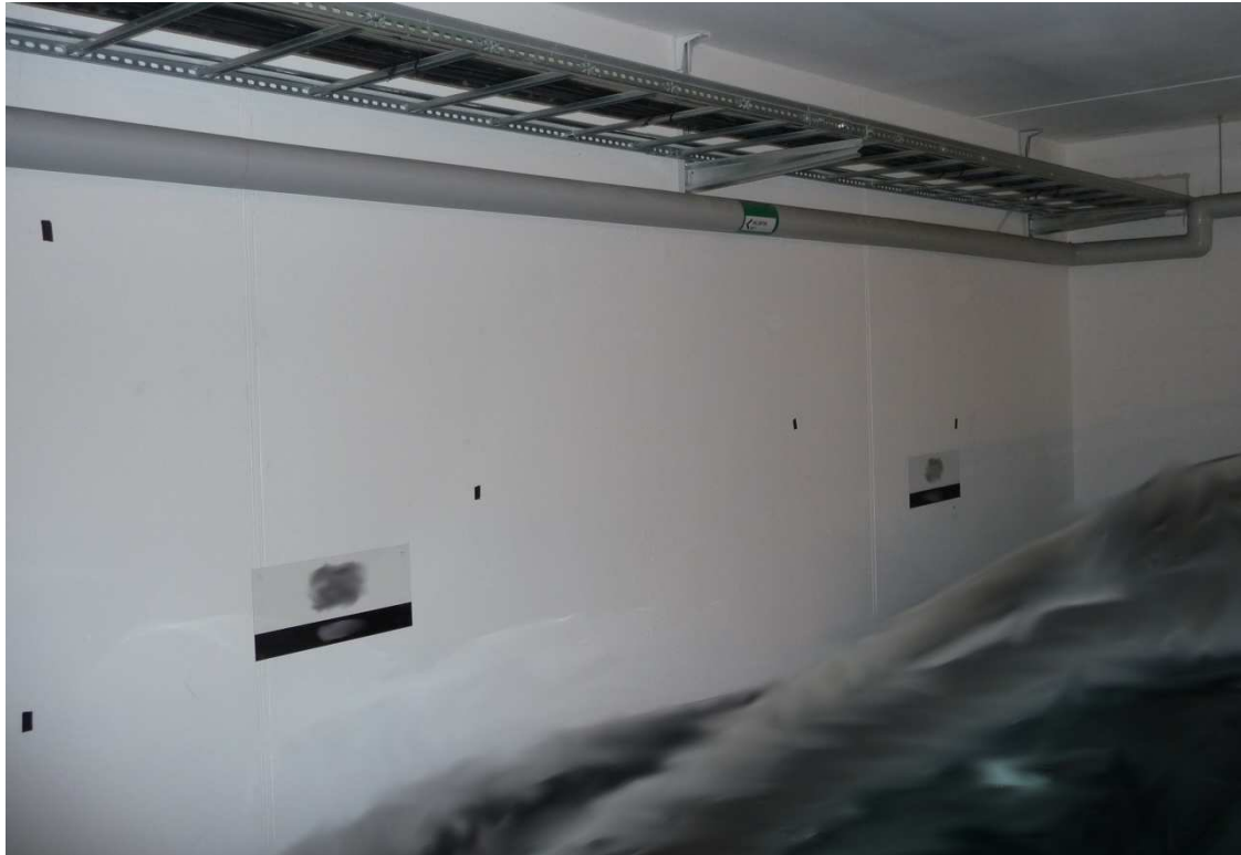
Figure 4.13 Overview of the left part of wall 2, object A
