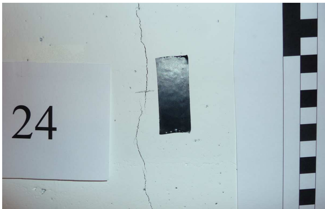
Figure 4.25 Example of crack in wall 1, object B
