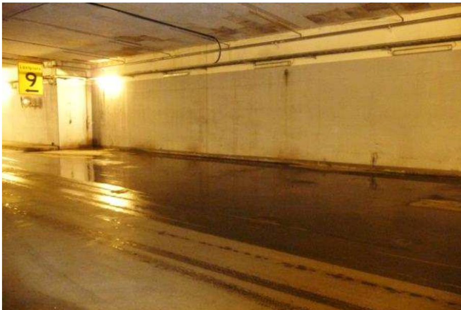
Figure 2.3 Water leakage in a cellar due to insufficient tightness
