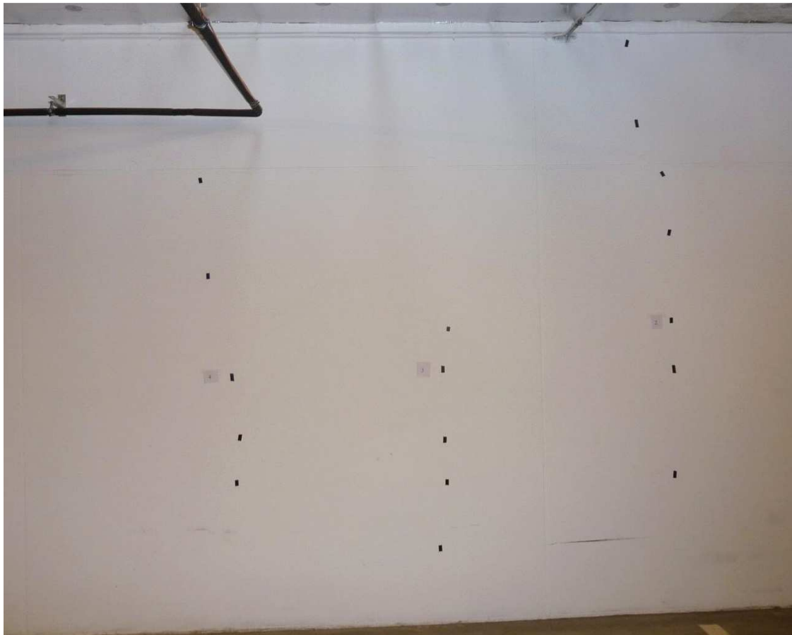
Figure 4.8 Closeup of cracks 2, 3 and 4 at wall 1
