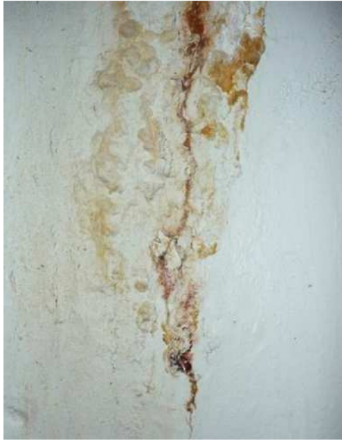
Figure 2.2 Discolouration near a crack caused by corroding reinforcement
