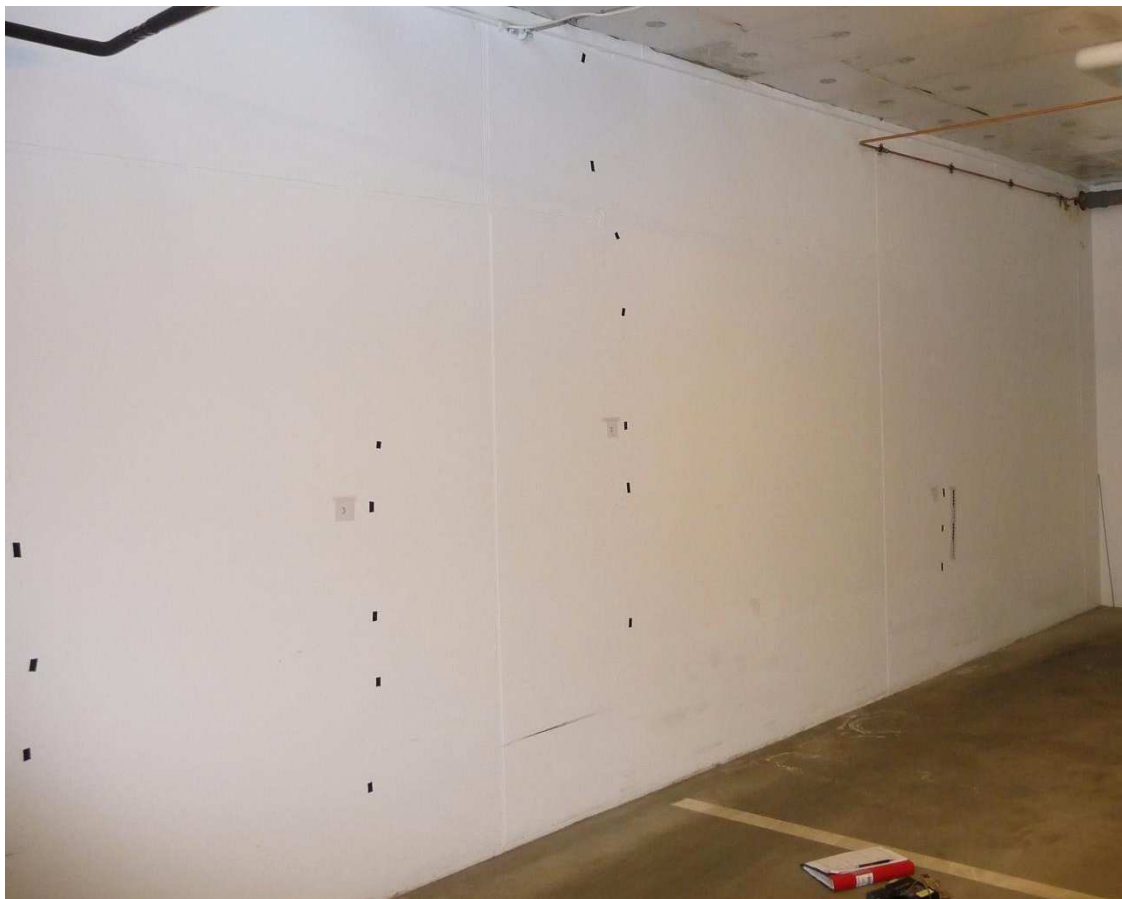
Figure 4.7 Closeup of cracks 1, 2, 3 and 4 at wall 1
