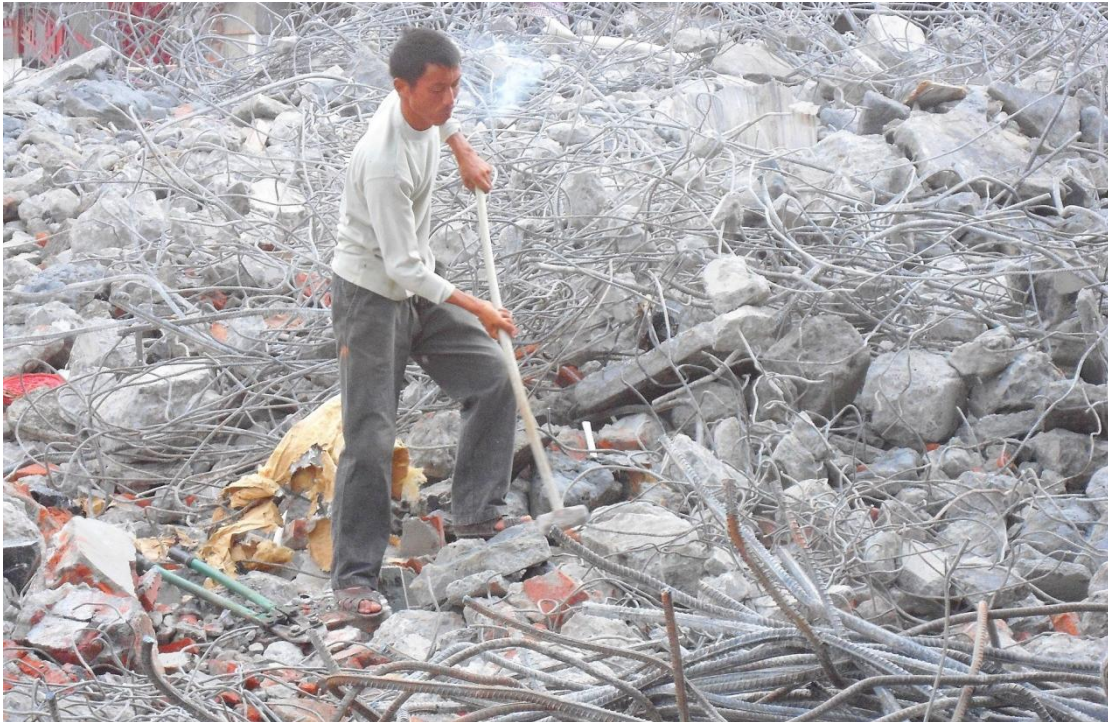
Figure 2 Retrieval of reinforcement steel from rubble (Frodesiak 2012).
