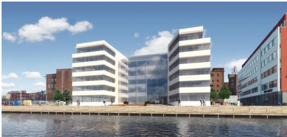
Figure 7 Aurora office building as seen from the river (Eklandia 2014).
