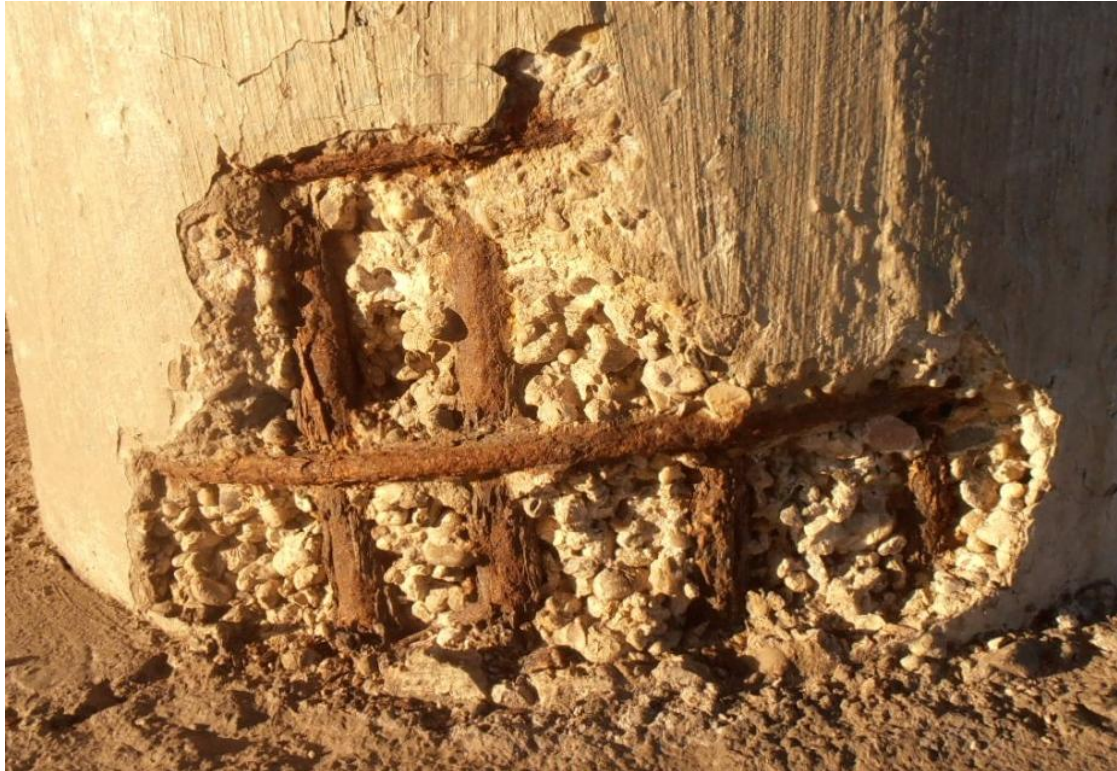
Figure 1 Concrete spalling (Sarang 2012).
