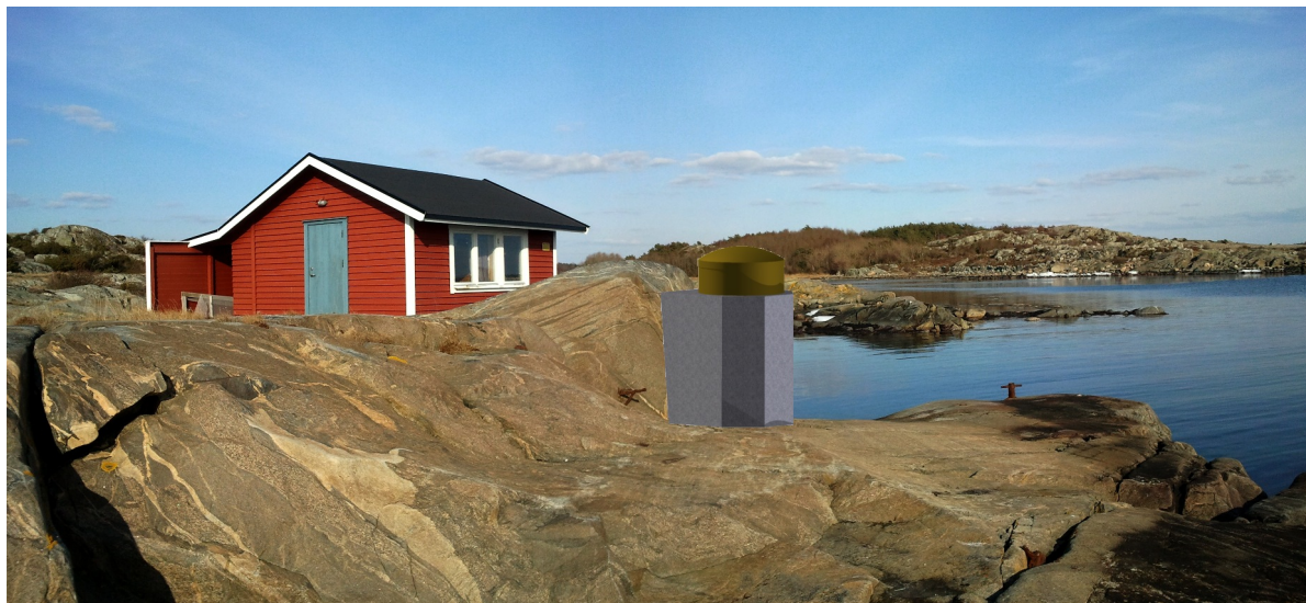
Fig. 5 An artist's impression of the planned official tide gauge station of the Swedish national network. The red hut exists and will be used to accommodate instrumentation for the tide-gauge station. A first preliminary installation is shown in Figure 4.
