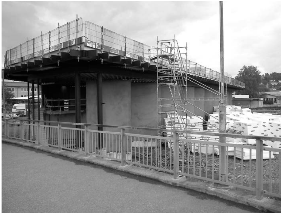
Figure 1. Bus terminal under construction (2011).
