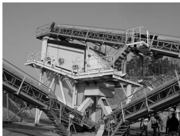
Figure 7. This screen is fed from the conveyor above coming in from the right. The products are then transported on different conveyor belts from the screen. NCC's Glimmingen operation, Uddevalla, Sweden (Photo E. Hulthén).
