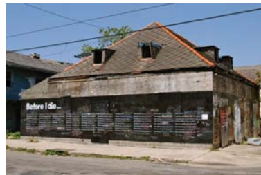
is clad with black boards with "Before I die.." printed on them..
