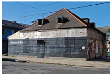
An abandoned building..
